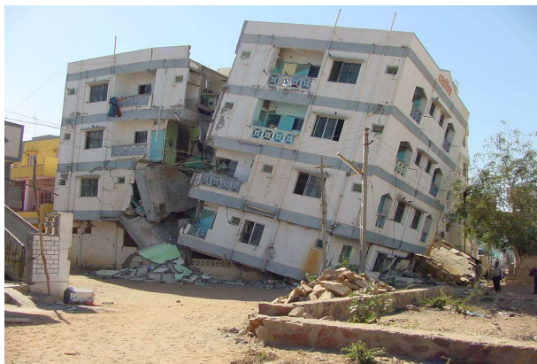
Soft Storey (Open Plinth), Vertical Split Between Two Blocks (Bhuj)
