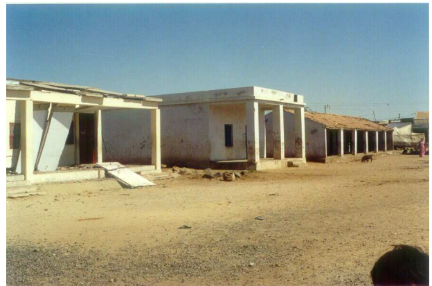
School roof with precast RC Panels collapsed (Gandhidham)
