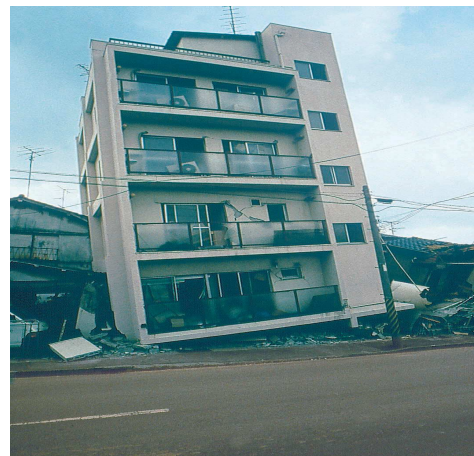
The well – braced upper part of the building collapsed onto the ground floor (Kachchh, 2001)
