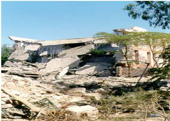
Government Hostel Collapse (Bhuj)
