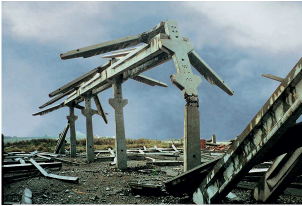
The consequences of bad planning & insufficient design & detailing of a prefabricated industrial building
