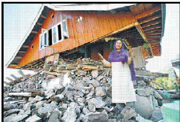
Destruction Due to Recent Earthquake in Jammu & Kashmir
