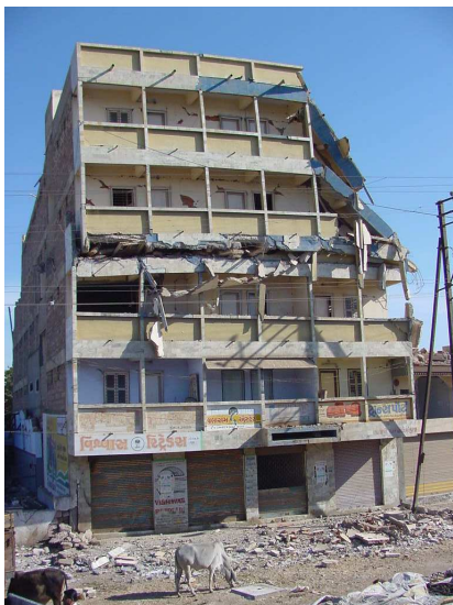
Soft Middle storey collapse (Bhuj)
