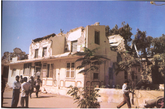
Collector Office at Bhuj Collapse of Second Storey
