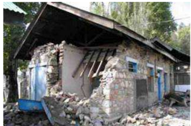
Collapse of Stone Masonry Walls
