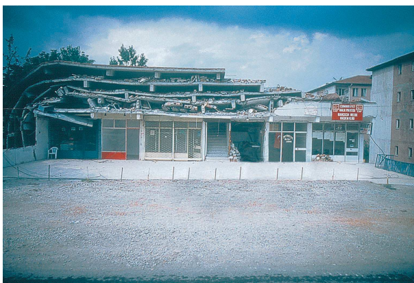
All the upper floors were too soft (Izmit, Turkey 1999)
