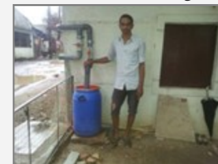
Rain Water Harvesting
