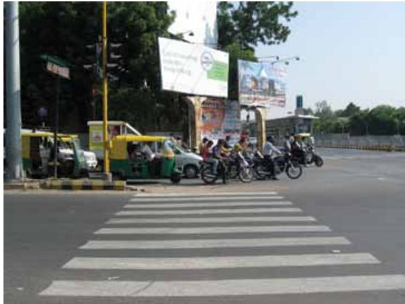
X Figure 2.22 This painted crossing is completely ineffective. Since drivers do not observe painted road markings, the only means of ensuring pedestrian safety is physical treatment, perhaps assisted by enforcement.
