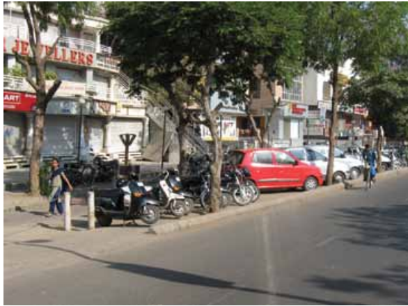
Figure 2.39 This street provides semi-formal parking areas that are accessed from a service lane. The design facilitates the collection of parking fees by delineating parking and no-parking zones and reduces the number of conflict points on the main carriageway.
