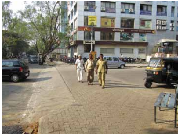
Figure 2.23 This raised pedestrian crossing compels vehicle users to slow down. The height of the crossing is the same as that of the adjacent footpath, improving convenience for pedestrians.
