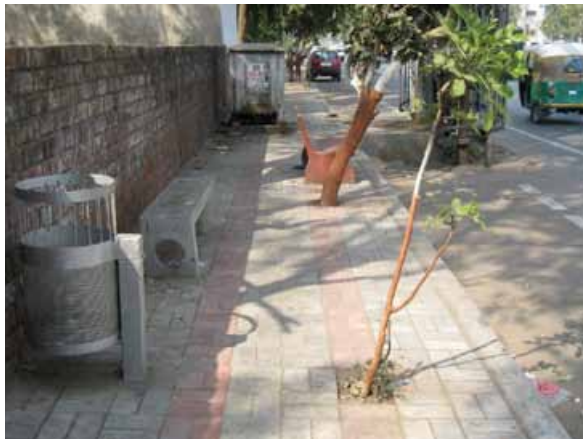
✗ Figure 2.2 This recently constructed footpath does not accommodate obstacles in a way that would allow pedestrians to effectively use the footpath.
