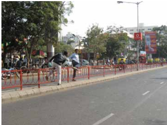
✗ Figure 2.20 This median fence is continuous, forcing pedestrians to climb over. There is no safe refuge, so pedestrians often stand in the carriageway while waiting for a break in the traffic.
