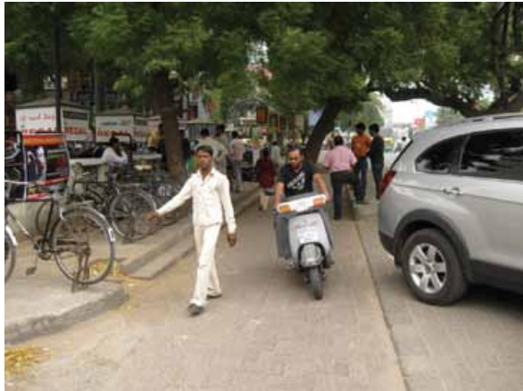
Figure 2.44 The narrow width of this service lane keeps vehicle speeds low and makes it a good shared space. While pedestrians have priority, vehicles can enter the service lane to access on-street parking and adjacent properties.
