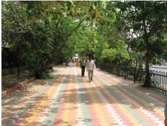
Figure 2.1 This footpath is wide, continuous, and shaded. However, the continuous fencing towards the carriageway prevents free pedestrian movement.
