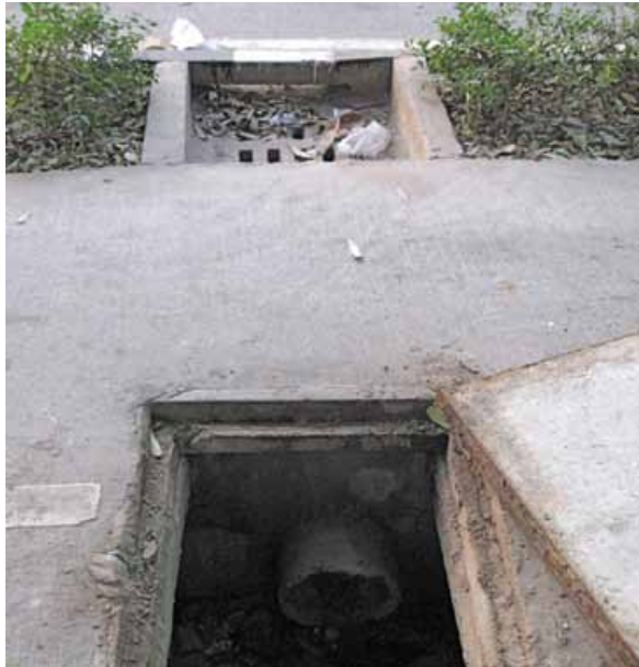
Figure 2.53 This design lets water fall into a catch pit in the buffer and then into pipes under a cycle track. The level of the drain is below that of the cycle track.
