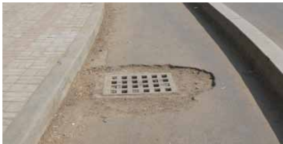
X Figure 2.54 The joint between the drain cover and the surface of a cycle track is substandard and the placement of the drain in the cycle track means that cyclists ride through the deepest water in the cross section.
