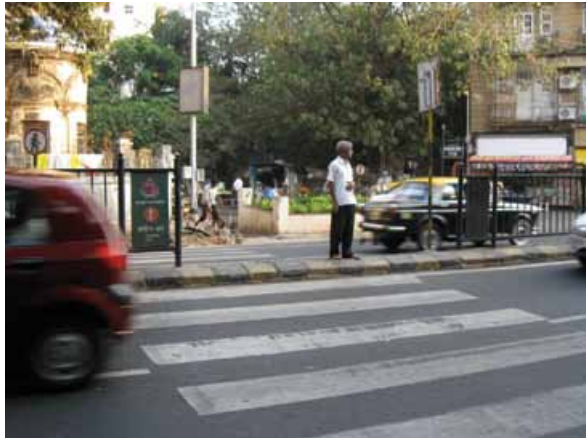
Figure 2.19 This opening in a median allows pedestrians to cross without climbing over the fence and waiting on the carriageway.
