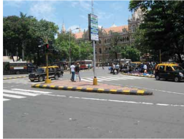
Figure 5.4 Existing left turn islands are fenced and landscaped. Instead of serving as refuge islands, they become barriers to pedestrian movement. Islands and medians will be redesigned to be accessible to pedestrians.
