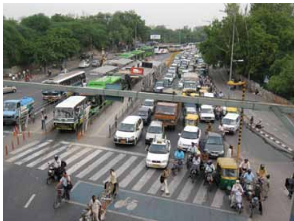
✗ Figure 2.13 BRT frees buses from traffic congestion so that they can provide prompt, reliable service. However, the width of this BRT station and its location directly at the intersection create unnecessary congestion, resulting in longer delays for bus riders and private vehicle users alike.
