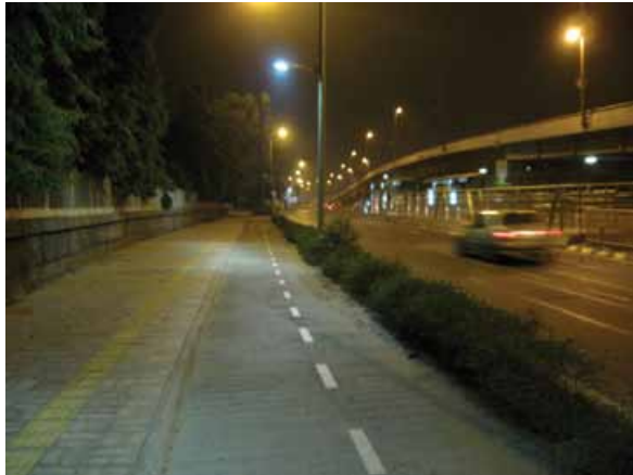
Figure 2.50 Good street lighting improves personal safety and reduces the risk of collisions. This street has sodium vapour lamps above the carriageway and metal halide lamps above the pedestrian footpath to ensure that the yellow tactile strip is visible to the visually impaired.
