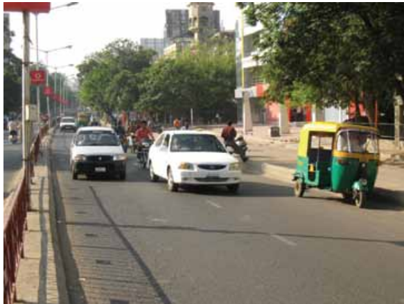
Figure 2.9 A properly scaled carriageway keeps vehicle speeds low and prevents wrong-way driving.
