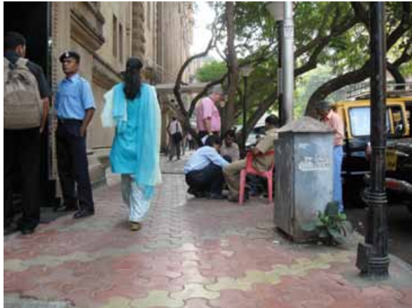
Figure 2.58 Utility boxes on footpaths should be oriented parallel to the street in order to maximise the free space available for pedestrian movement.
