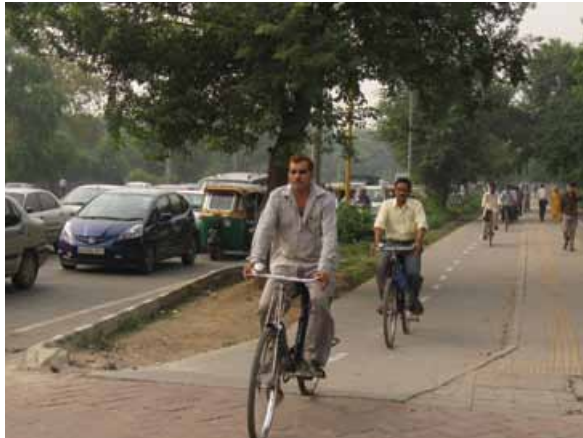
Figure 2.6 This cycle track is continuous and shaded. Curb heights are appropriate, and storm water drains into catch pits located in the landscaped buffer.
