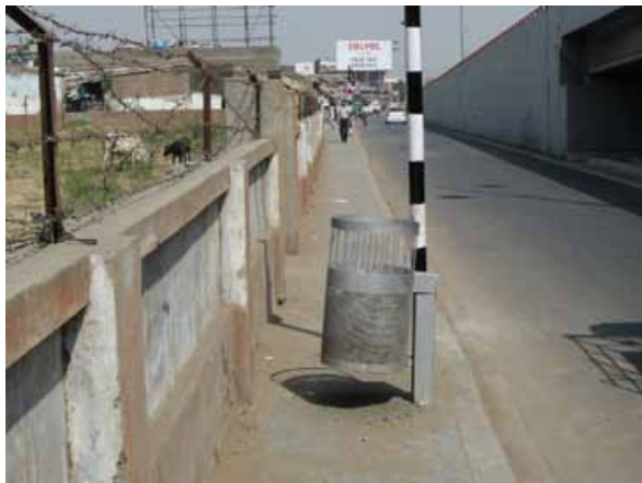
✗ Figure 2.36 Street furniture should be positioned so that it does not obstruct pedestrian and cyclist movements. This garbage can makes it impossible to continue walking on the footpath. If such obstacles are frequent, pedestrians will not use footpaths at all.
