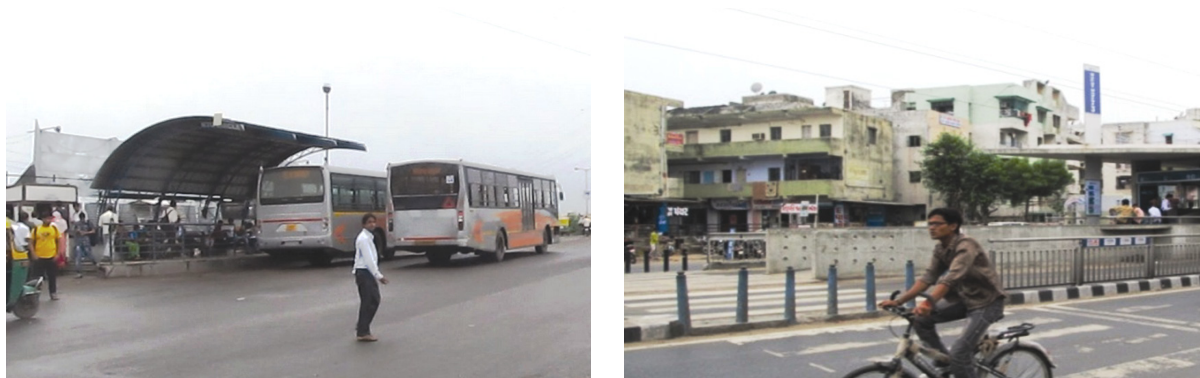
Figure 4.20 (Left) R.T.O. bus station: Low height, no ramp, no level boarding (Right) Concrete pillars at entry of station
