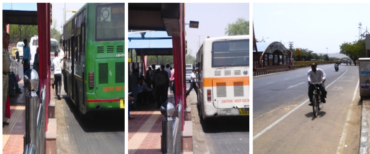
Figure 3.34 (1) Level-boarding problems (2) Bus distanced from the platform (3) Cycle track
