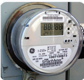
Smart electric meter
