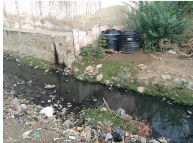
This picture shows the temporary method of treatment applied for drains that carry sanitary discharges. Local O&M staff refer to this treatment method as bioremediation (not the proper name in the US tech terms). It is expected to reduce BOD<sub>5</sub> from 80 to 30 with this bioremediation. No data is available if this system effectively reduce biodegradable material in the wastewater.
