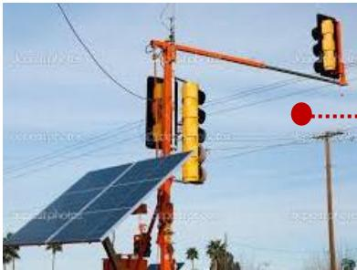
**SOLAR TRAFFIC LIGHTS POWERED BY SOLAR PANELS AT ROAD INTERSECTIONS, PEDESTRIAN CROSSINGS ETC.**
