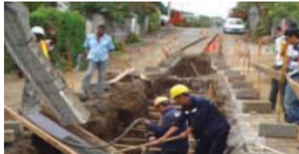
Construction of sewerage system. (Source: IWA)
