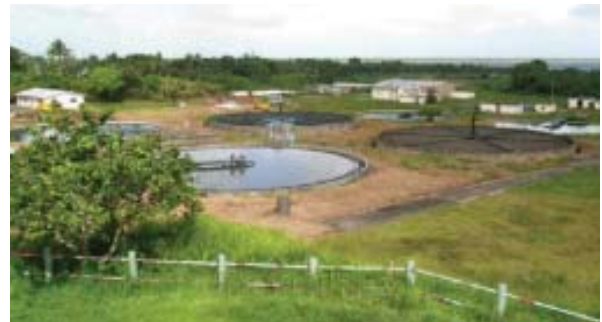
sequential batch reactors (Source: ADB)
