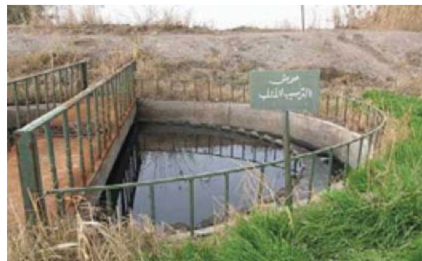
Sedimentation Tank (Source: IWA)
