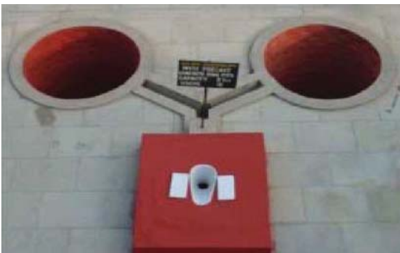
Sulabh Two-Pit-Pour-Flush Toilet (Source: B. Pathak)
