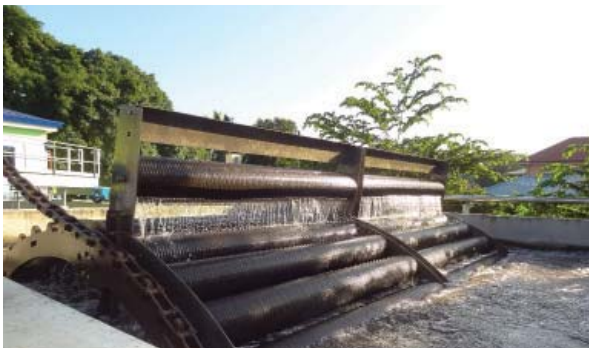
STM Aerotor (Tandang Sora STP) (Source: M. Ebarvia)
