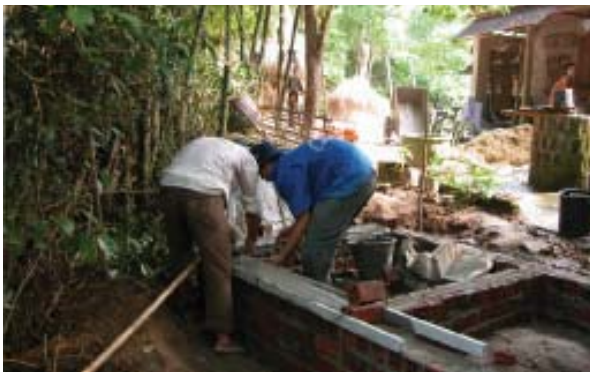
Construction of toilet and septic tank (Source: Do Nhat Hoang)
