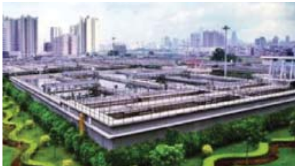
Liede sewage treatment plant (Source: Lin Duan)
