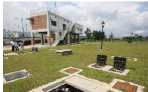
Olandes STP (Marikina City): process tanks built underground and support facility on stilts (Source: Steve Griffiths)
