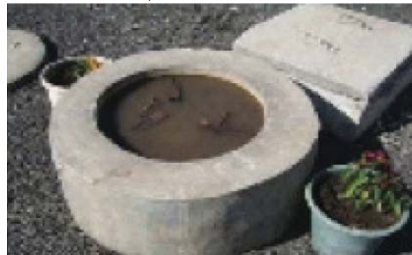
Area of top manhole, above the biogas fixed dome (Source: SuSanA)
