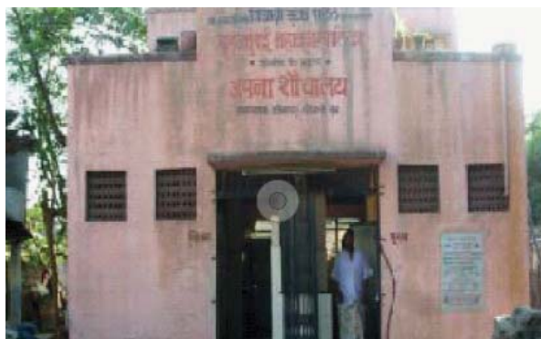
Toilet block (Source: Water and Sanitation Program)
