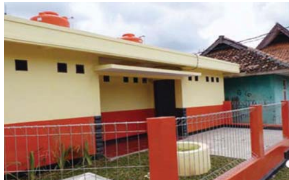
Community toilet block with biogas digester (Source: RTI International)
