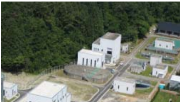
Aerial view of the Suzu City wastewater treatment facility. (Source: Saburo Matsui)
