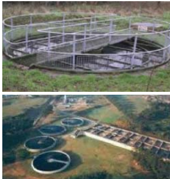
Wastewater treatment plant in Durban (Source: IWA)
