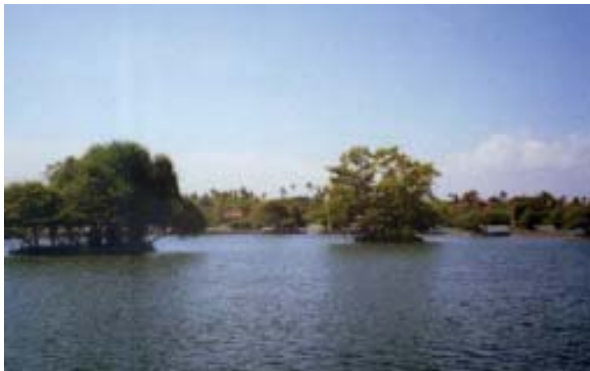
Wastewater treatment ponds: “Eco-Lagoon” (Source: M. Ebarvia)
