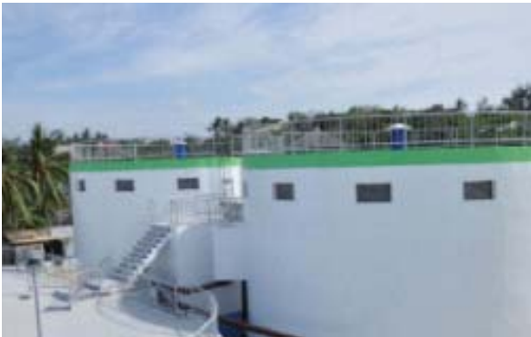
Boracay Island Water Company (Source: Bernardo Mañosca)
