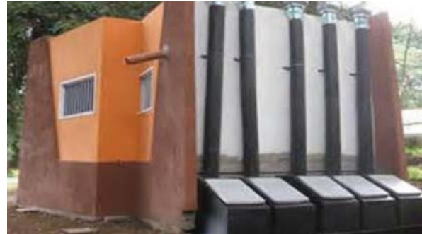
Ikotoilet urine-collection system, City Park, Nairobi, Kenya ( http://bit.ly/1ixvF7z )
