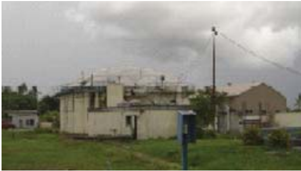
anaerobic sludge digester (Source: ADB)
