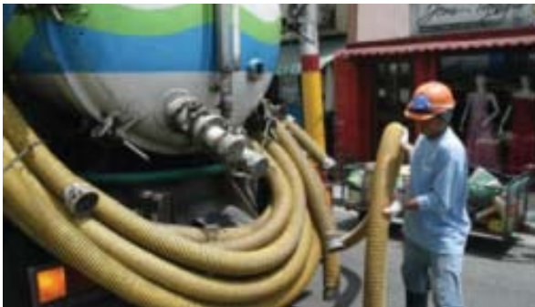
Vacuum trucks for desludging septic tanks. (Source: S. Griffiths)
