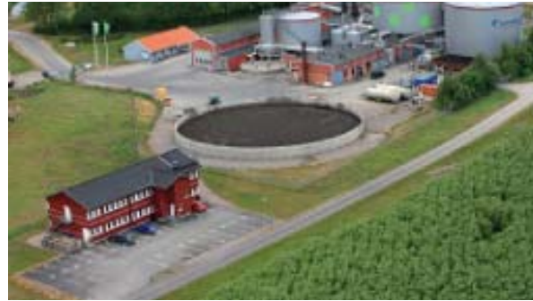
Linköping biogas plant (Source: Svensk Biogas)
