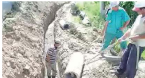
Construction of small-bore sewer system (Source: UNV/Natasha Mistry).
