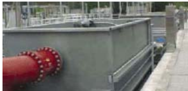
Orange County wastewater treatment plant (Source: IWA)
