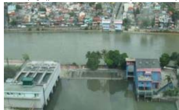
Poblacion STP (Makati City): elevated and on top of a Flood Control Pond (Source: MWCI)
