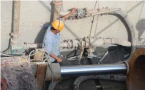
Sewerage construction (Source: ADB)
