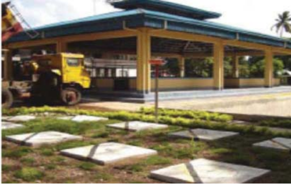
View of the anaerobic treatment modules: settling tank (ST), anaerobic baffled reactor (ABR), and anaerobic filter (AF). (Source: BORDA)
