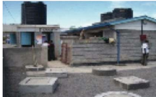
Sanitation facility with water kiosk. Underground biogas plant in front (Source: Sustainable Sanitation Alliance)
