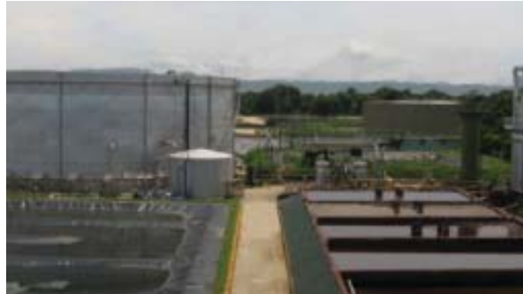
Thermophilic anaerobic digester and lagoons (Source: G. Tee)
