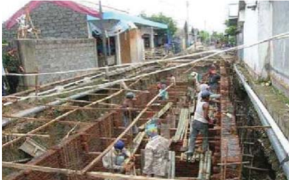
During construction (Source: Yuyun Ismawati)
