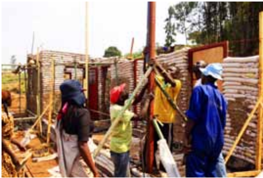
FIGURE 44: EARTH BAG CONSTRUCTION
