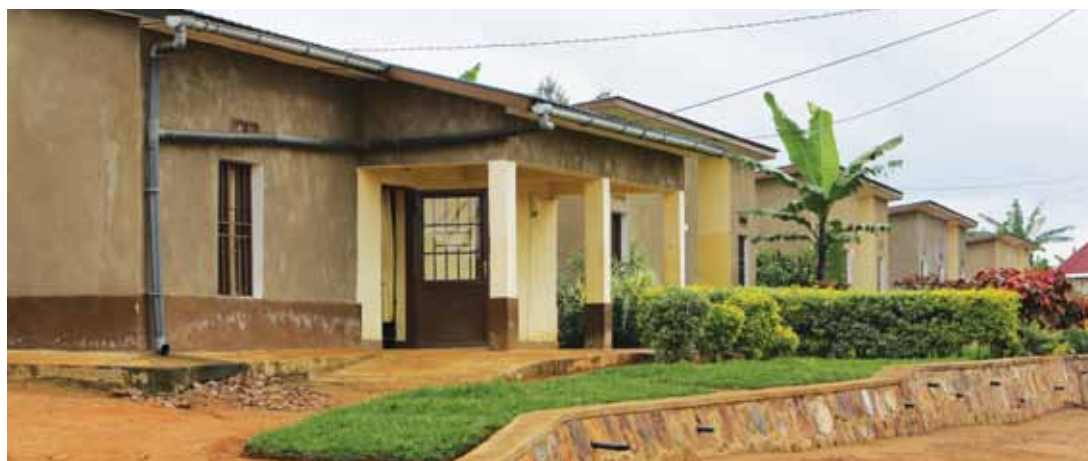
FIGURE 40: LOW WINDOW AND EXTERNAL DOOR WITH GLAZING TO ALLOW VIEW FROM WHEELCHAIR
