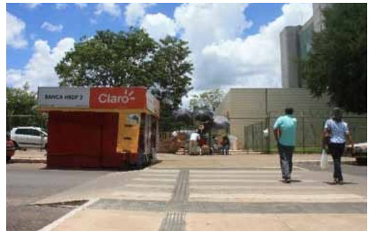
FIGURE 10: ELEVATED PEDESTRIAN CROSSING, BRASILIA, BRAZIL
