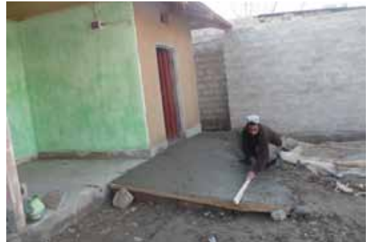
FIGURE 48: NOOR JEHAN HOUSE, (RAMPED ACCESS UNDER CONSTRUCTION)
