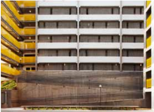
FIGURE 43: RAMPS AND STREET VIEW
