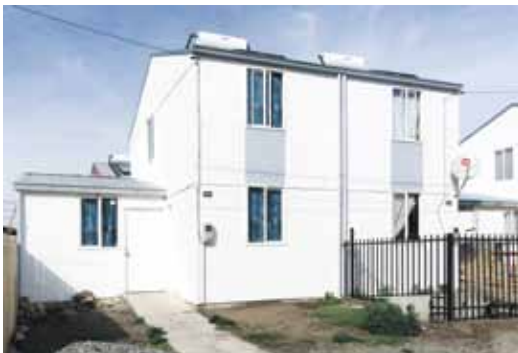
FIGURE 53: ADAPTED HOUSES WITH SHW SYSTEMS
