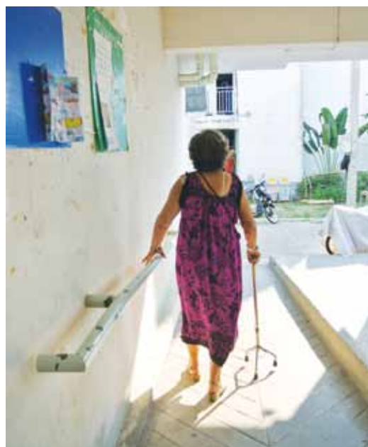
FIGURE 54: TYPICAL RESIDENTIAL BUILDING IN BAAN EUA AR-THORN. RAMPS AND HANDRAILS WERE PROVIDED IN EVERY BUILDING
