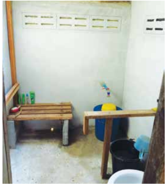
FIGURE 56: (RIGHT) TOILET IMPROVEMENT WITH HANDRAILS AND BATH CHAIR
