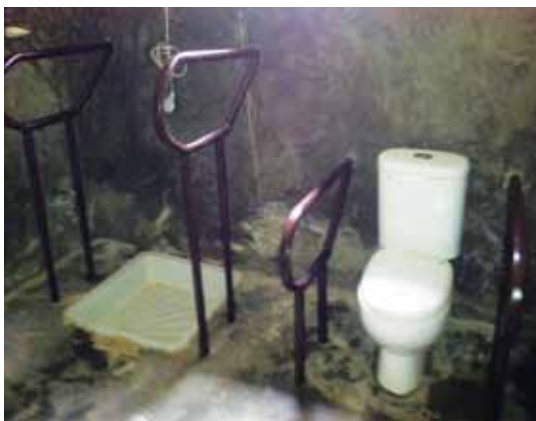
FIGURE 39: BARRIER FREE WASHROOMS
