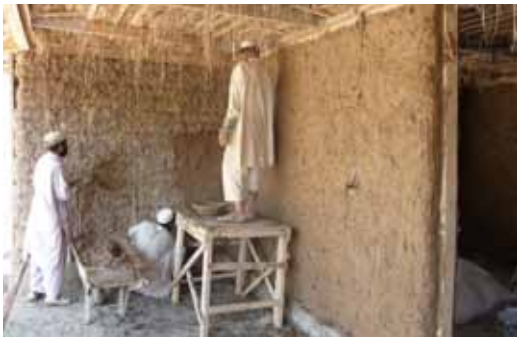
FIGURE 47: NOOR JEHAN HOUSE, (EXPOSED STRAW BALE UNDER PLASTER)
