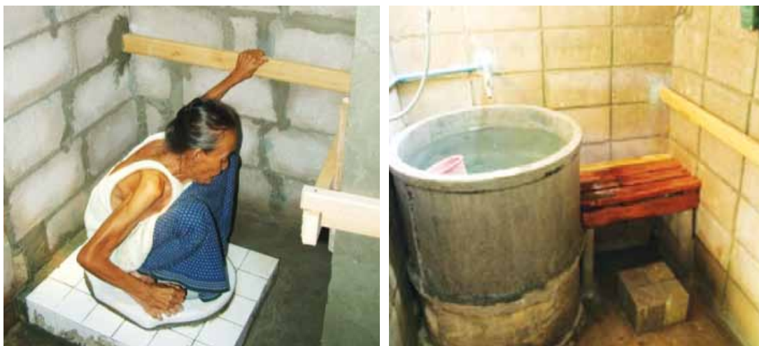
FIGURE 57: FLAT TOILET AND BATH CHAIR PROVISION WITH HANDRAILS
