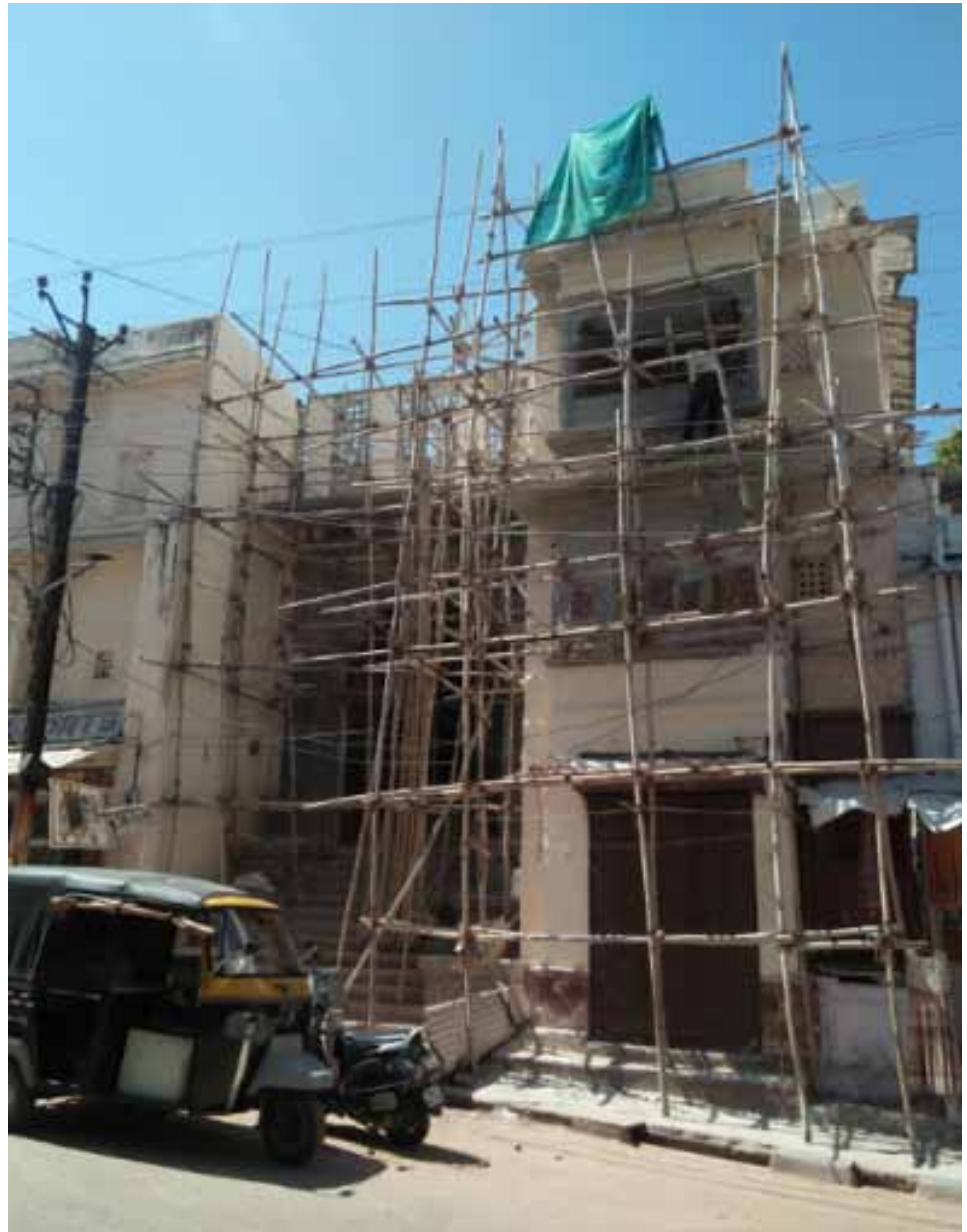
Ongoing conservation work of bazaars in the Walled City area
