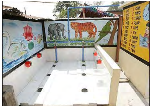
Children-friendly community toilet.
