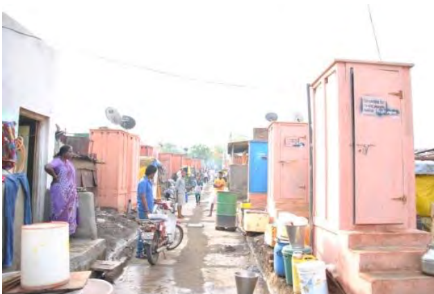
Vita: Two ODF slums in Vita though infrastructure provision by the ULB.
