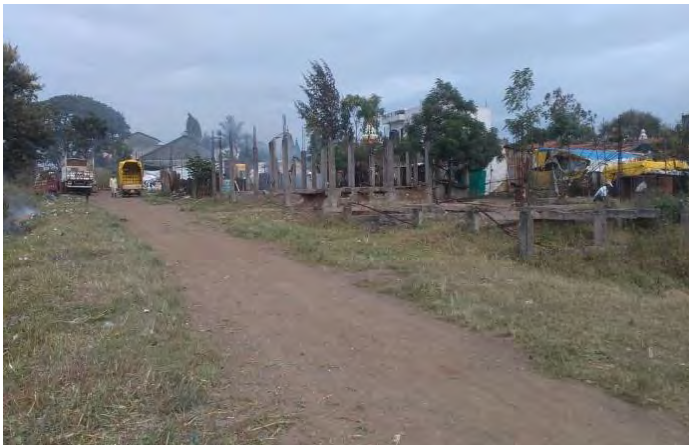
Kagal: Construction site of a community hall which is being developed on an OD spot.
