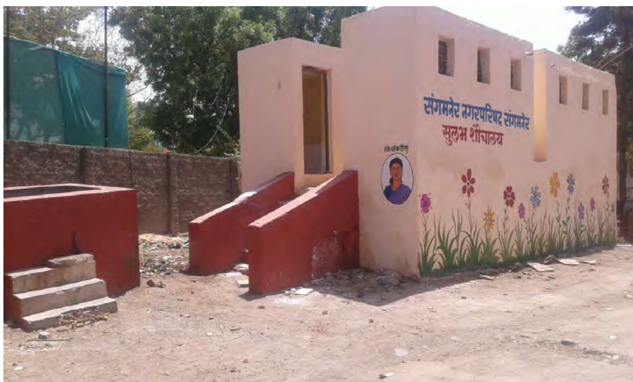
Sangamner: Newly constructed community toilets.
