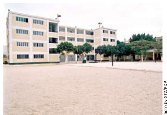
Upgrading of schools
