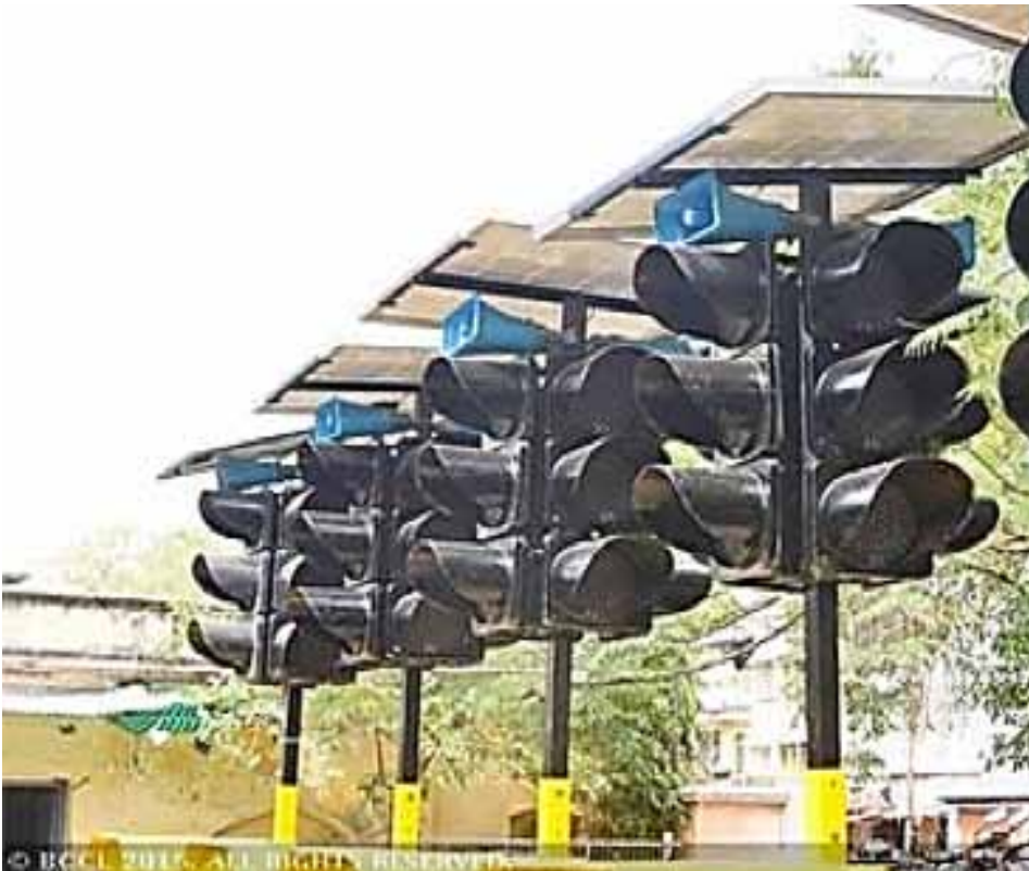
Adaptive Traffic Signal Control System – Bhubaneswar
