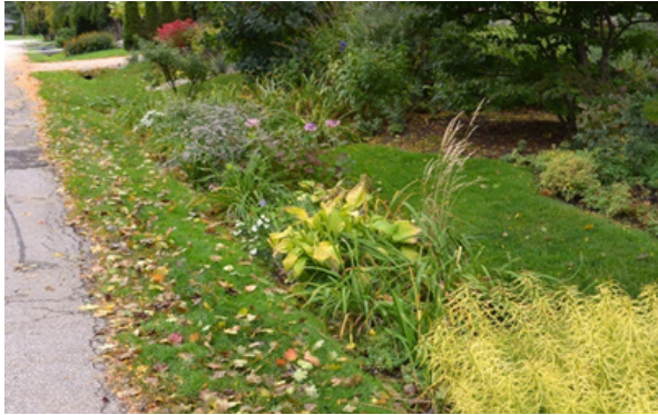
Image 25 | Swales created on the edge of the road with local vegetation
