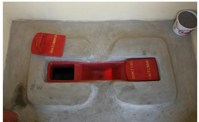
**Fig. 8:** Inside view of a UDDT with ash container on the right. The squatting pan has two faeces outlets: only the one on the left is currently in use. In the left corner is the ventilation pipe (not visible) (source: Moses Wakala, GTZ-Kenya, June 2008).
