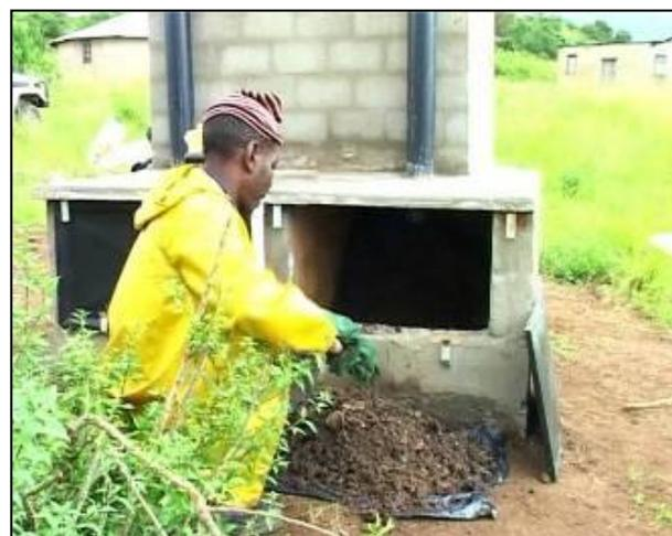
**Fig.14:** Emptying a UDDT faeces chamber (source: EWS.).
