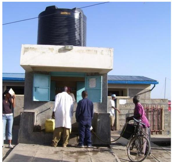
**Fig. 5:** Customers of the water kiosk. The water tank on the roof holds 5 m<sup>3</sup> (or 250 jerry cans) to bridge water supply gaps for a period of about 1-2 days.
