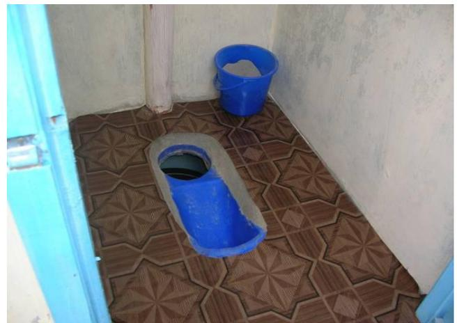
**Fig. 6** Inside the single vault toilet at the church showing the urine diversion pedestal and a container of ash.
