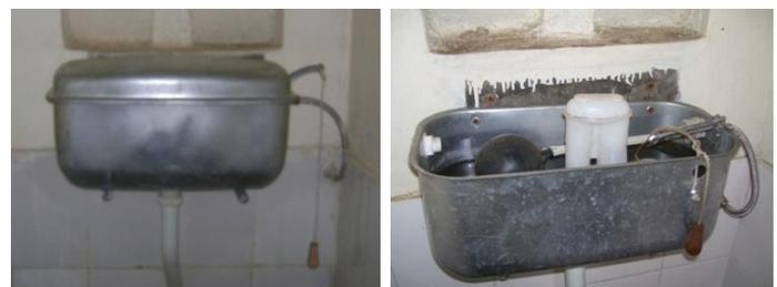
Fig. 13: Cistern after installation (left) and after vandalism/misuse and theft (right) a few weeks later. Repairs were undertaken by WSP, but the toilet operator now shifted to a pour flush system.
