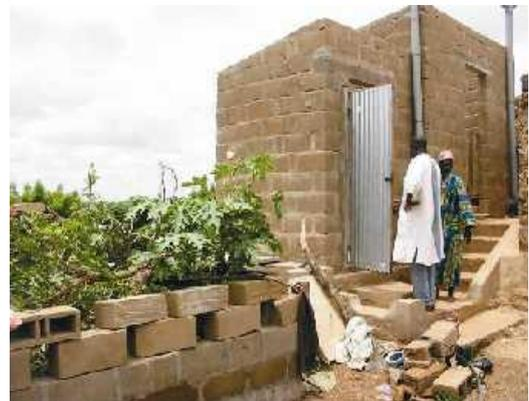
Fig. 3: Ecosan UDD toilet in Koulikoro with shower and greywater garden in 2002 (source: GTZ, 2002).
