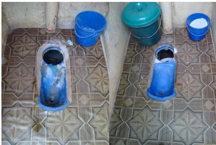
**Fig. 14** On the left, inside view of toilet used by men with empty ash container, urine on the floor and signs of faecal cross-contamination. Right: Inside view of toilet used by women (Source: L. Kraft, May 2011)
