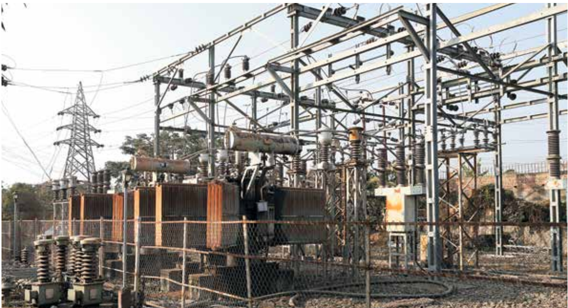
Karong substation in Senapati District
