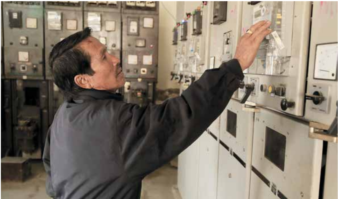
An employee at work at Karong substation in Senapati District
