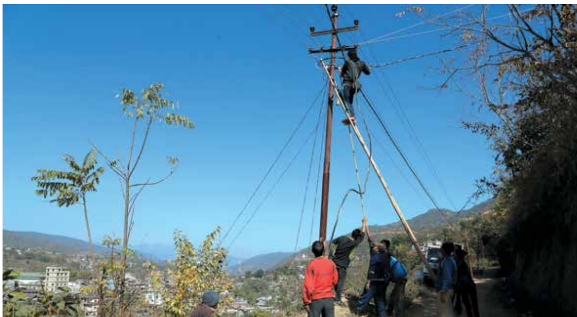
Linesmen stringing the Aerial Bunch Cable (ABC) in Senapati District
