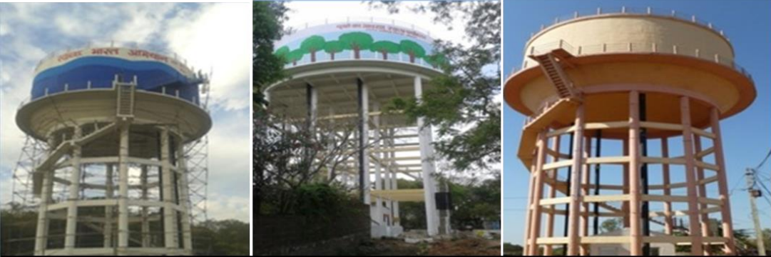
Bhopal Water Supply Infrastructure
