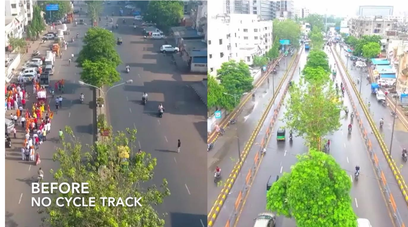
Visually Improved, congestion free & Safer Roads; Improved road junctions
