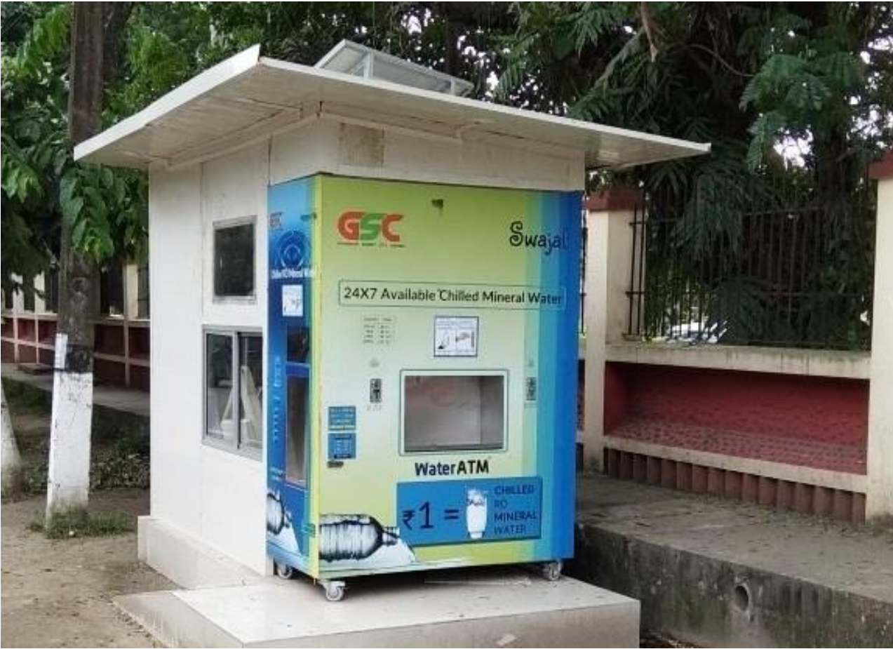
Guwahati Water ATM at Regional Center, Khanapara – Automated Water Dispensing Units to provide safe drinking water to floating population (at 20 locations)
