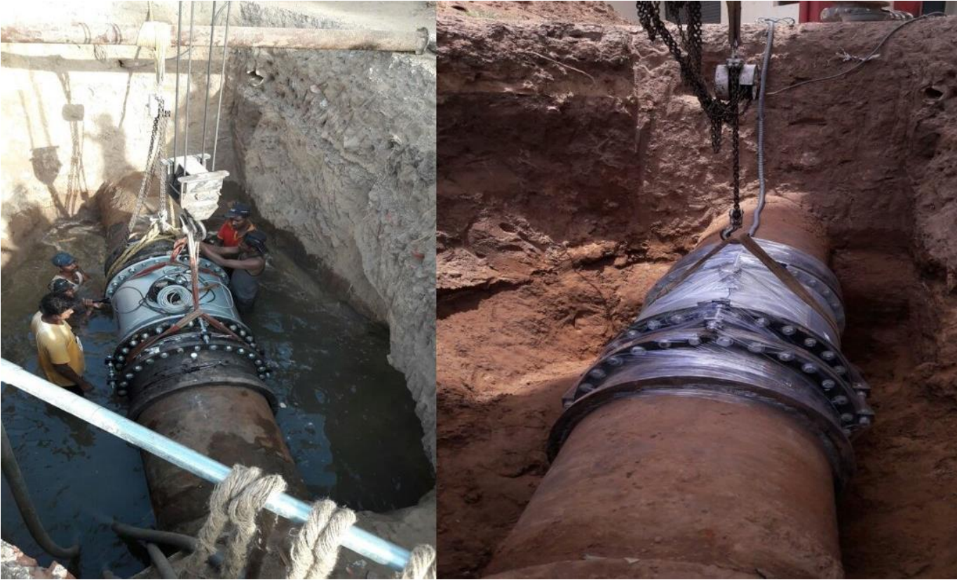
Ahmedabad – Effective water supply operations with SCADA implementation
