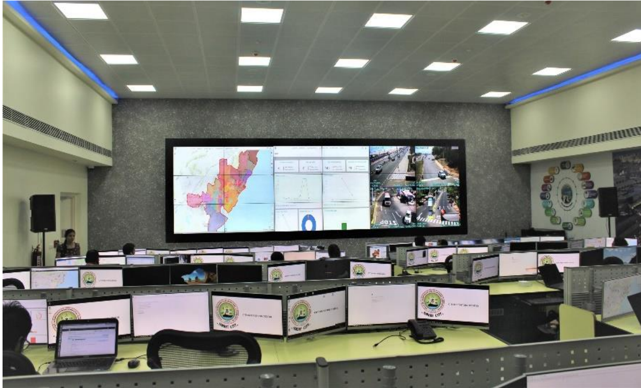
Visakhapatnam ICCC - Smart Poles & Environmental Sensors at 50 locations monitor real-time pollution
