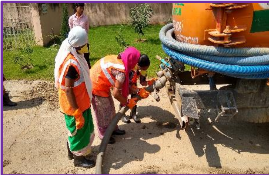
Women SHGs desludging at the sludge receiving chamber at Sambalpur SeTP
