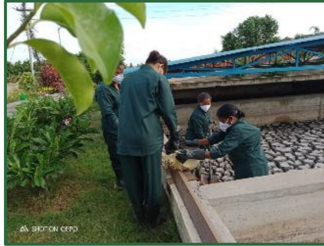
Women SHGs removing dried sludge cakes from the Sludge Drying Bed
