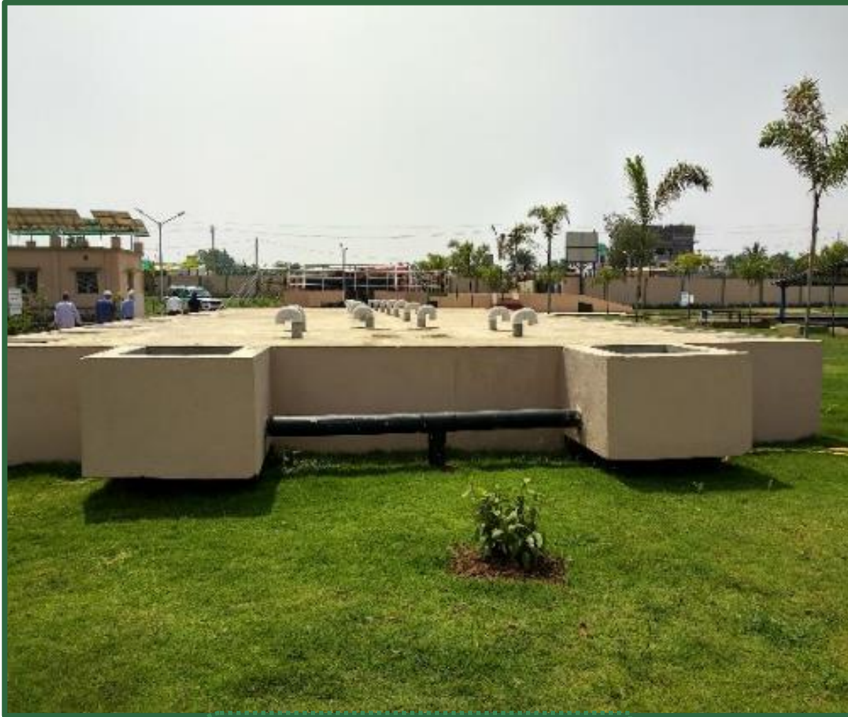
Anaerobic Baffle Reactor
