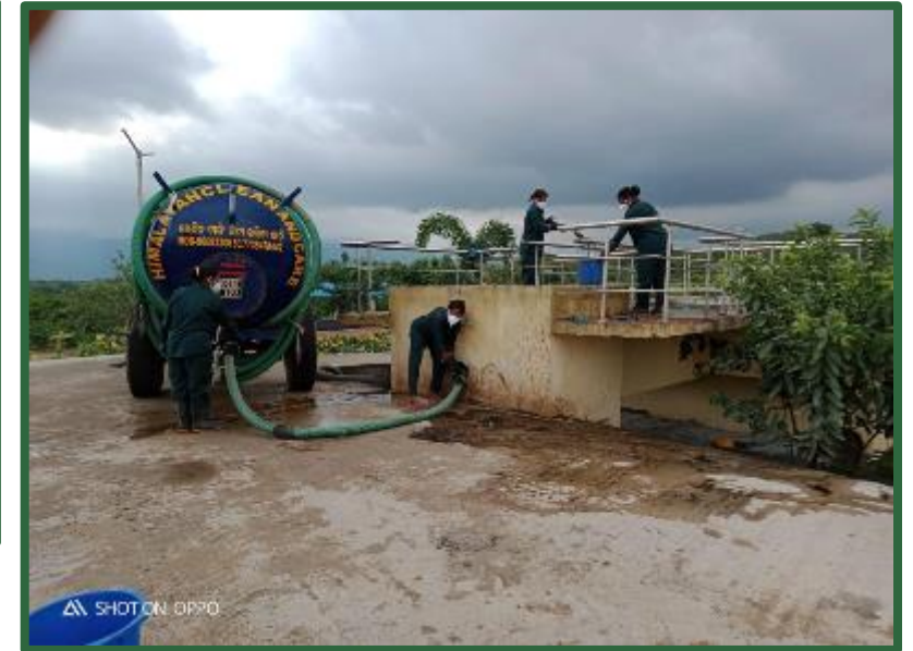
Women SHGs desludging at the sludge receiving chamber at Berhampur SeTP
