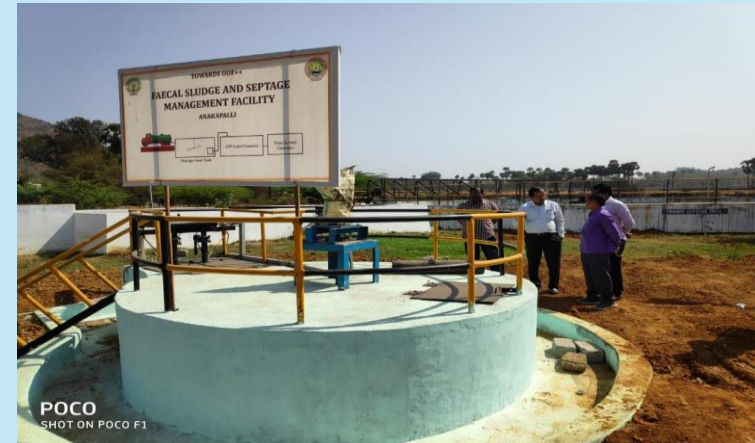
Co-treatment facility at Anakapalle STP
