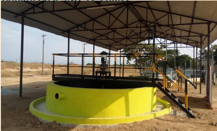
Co-treatment facility at Tirupati STP
