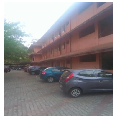
Figure 6.15 New PG Hostel
