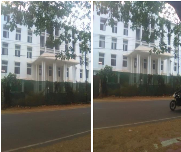
Figure 6-24 PWD building under construction
