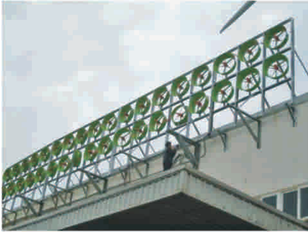
■ Factory Energy Saving
