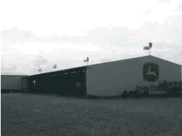
■ Factory Energy Saving
