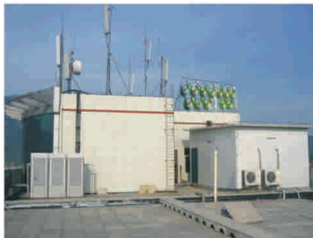
■ Power for Base Station
