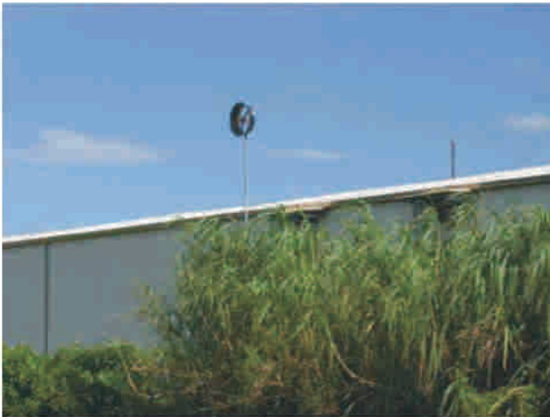
■ Factory Energy Saving
