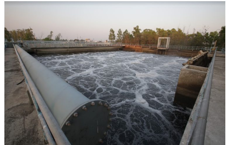
STP at Coimbatore
