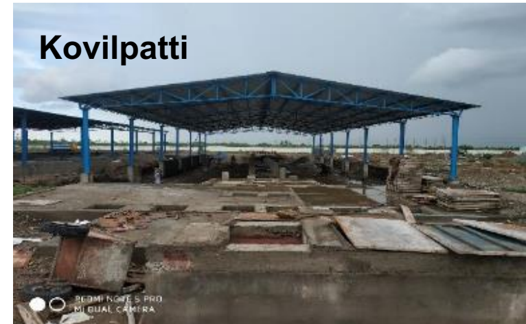
SDB-01: Floor PCC laying work is in progress
