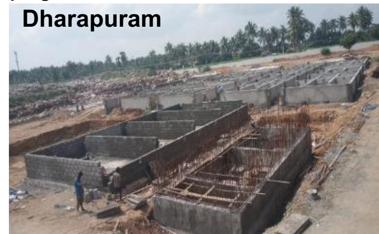
ISAF: Wall concreting is in progress
