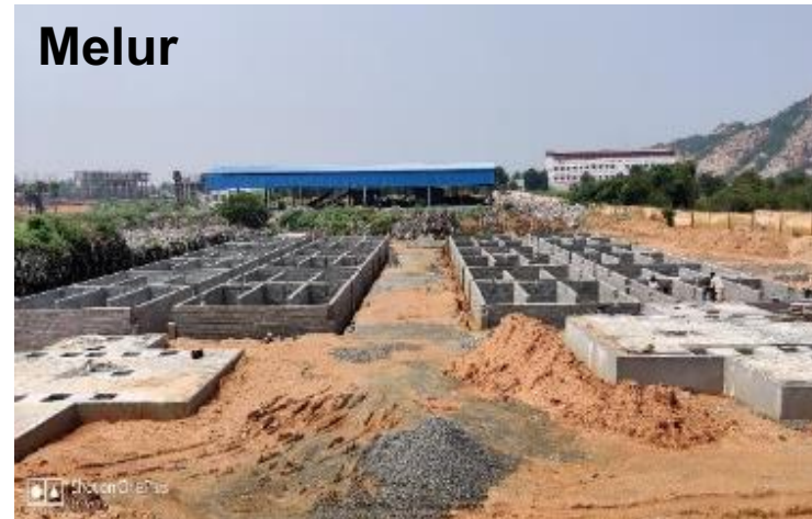
SDB-02: Plastering work is in progress
