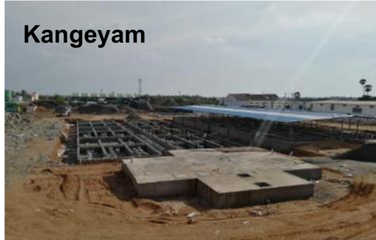
SDB-02: Finishing works are in progress
