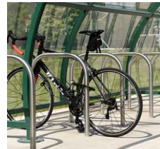
Ref. Image :SS Bicycle stand fixed over Concrete Base at Gate 1
