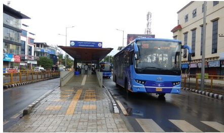
Well developed PT System
