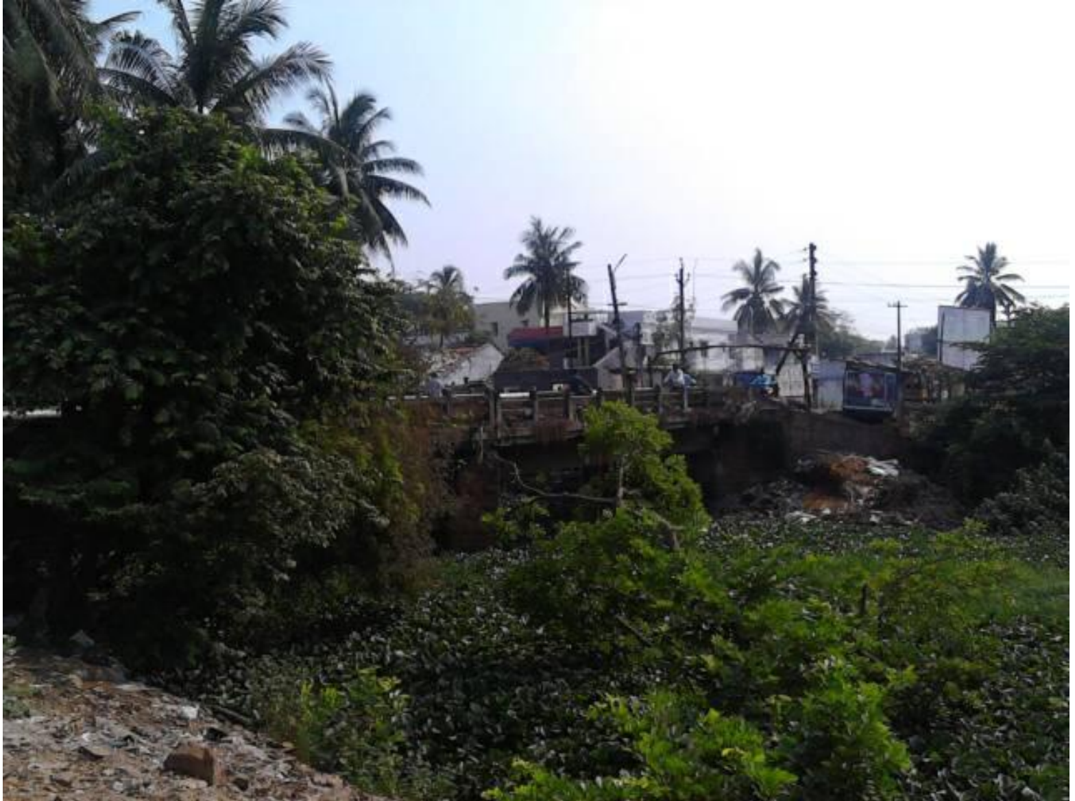
Plate 7: Site available for cross bund formation for temporary diversion of traffic and drain water
