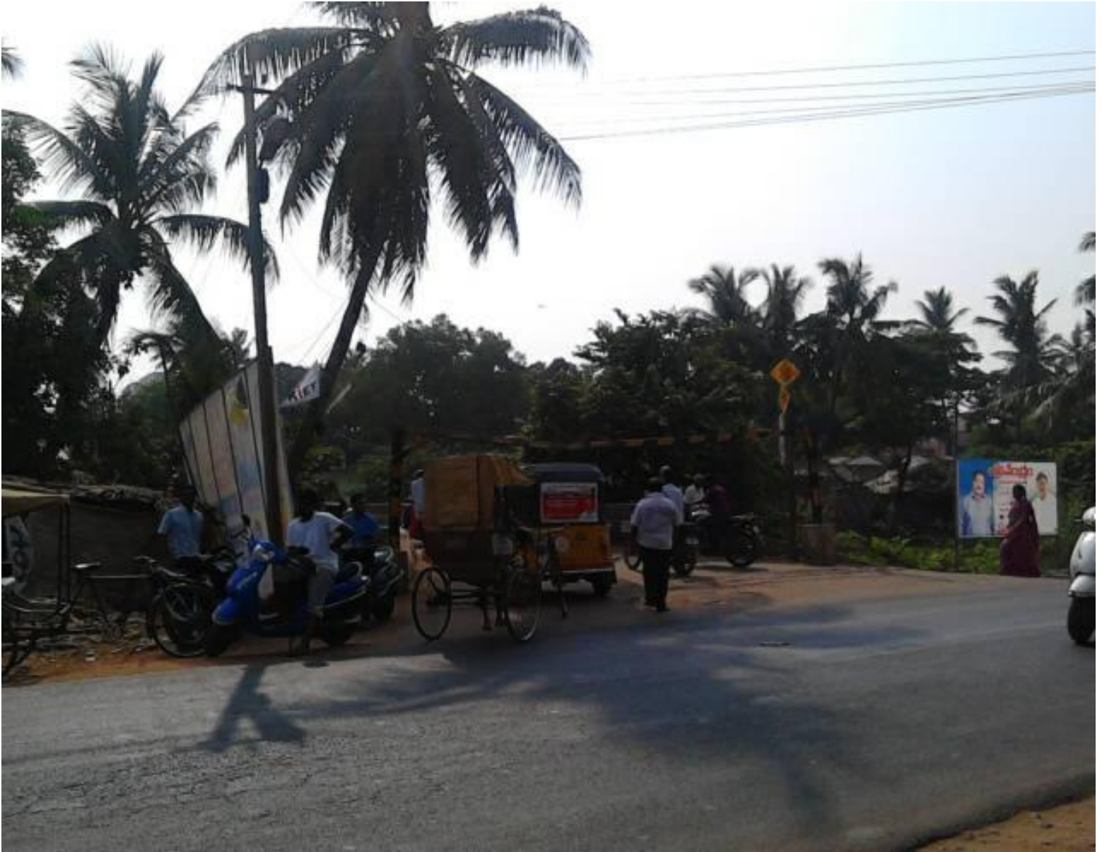
Plate 6: View of Kakinada-Samalkot Road - entry of traffic flow into proposed bridge
