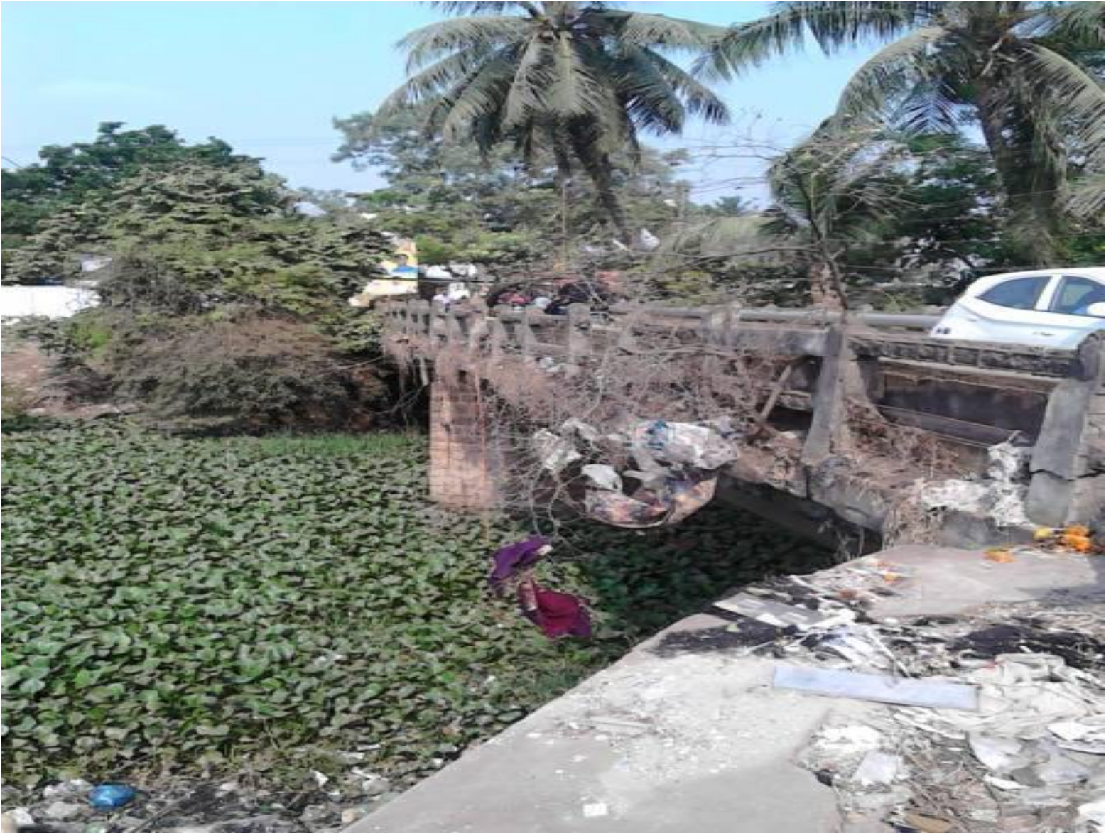
Plate 5: Drain flow and existing old bridge under normal flow conditions – need to have vacuum dewatering system for foundation concrete laying
