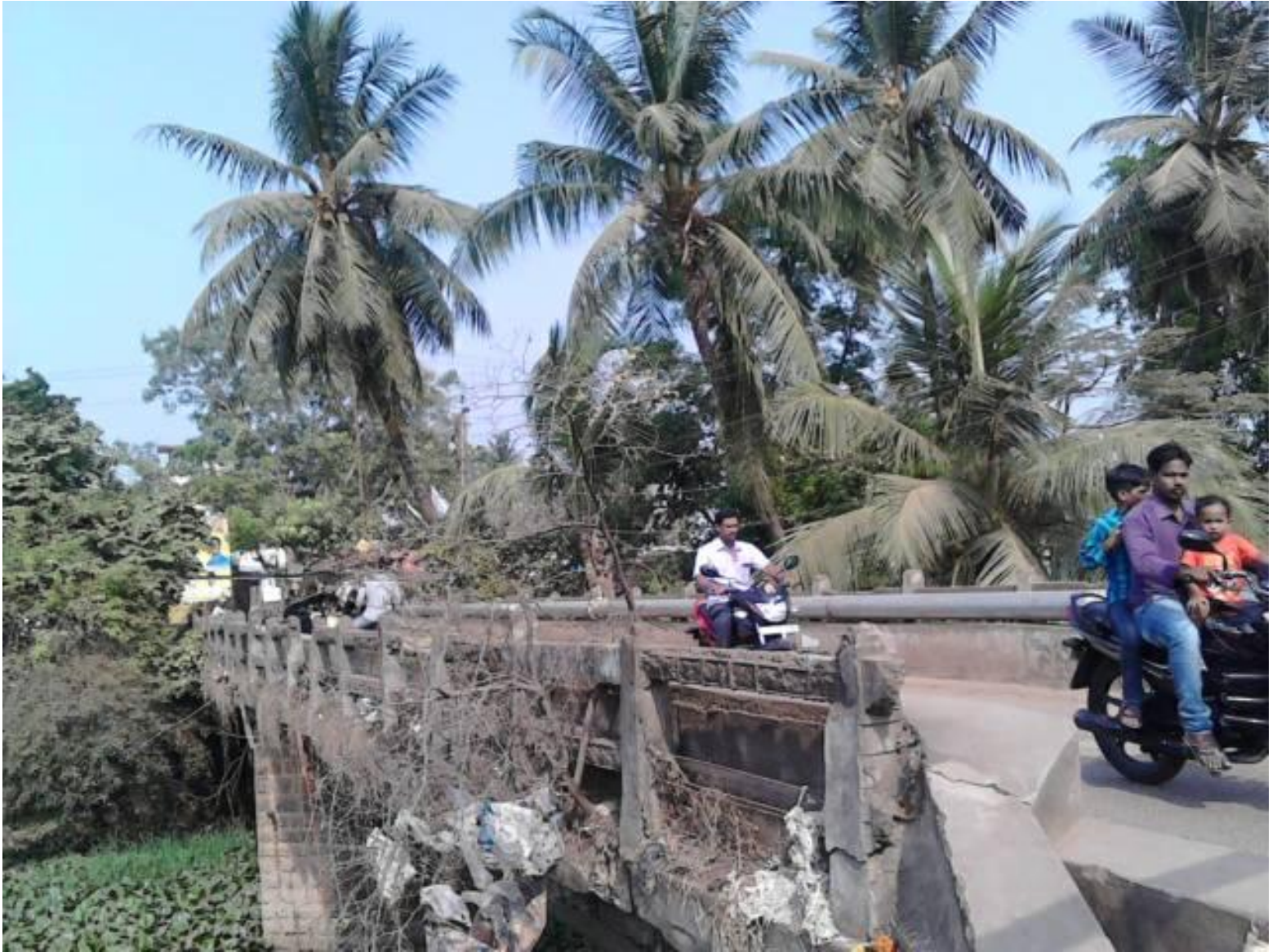
Plate 4: Existing single lane bridge to be dismantled during proposed bridge construction
