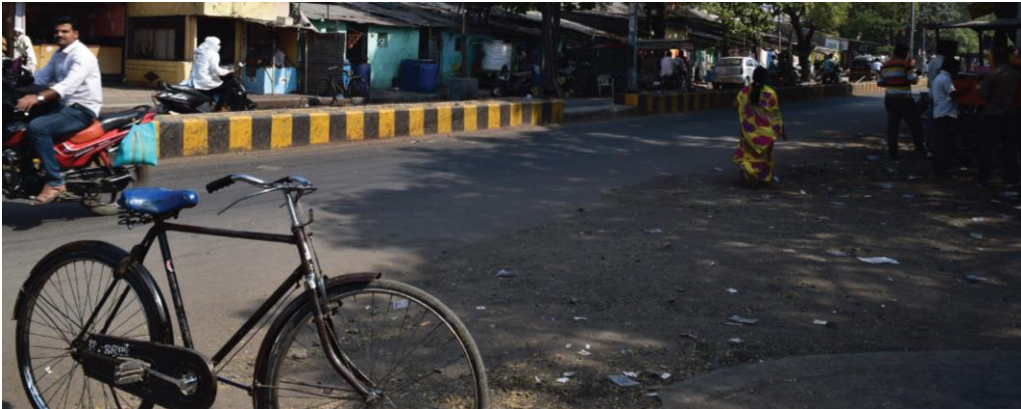
Figure 4 Undefined road edges
