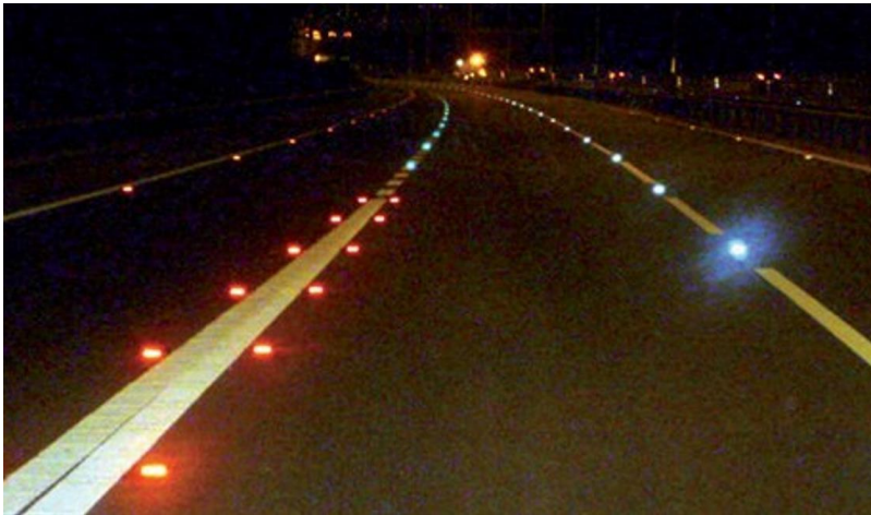
Figure 16 Raised pavement markers installed along road edges
