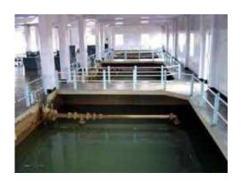
The entire bed should be taken out and additional sand mixed to give the required effective size and uniformity coefficient. Before starting the filter, the sand has to be backwashed to stratify the bed.
