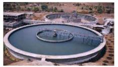
As well as problems from sludge build-up. Outlet weirs should be kept cleaned at all times. Algaecide or bleaching powder may be used for controlling biological growth on weirs.
