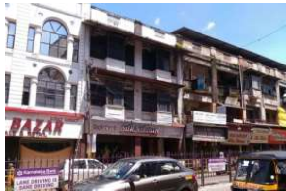
Road frontage on Balmatta Road
