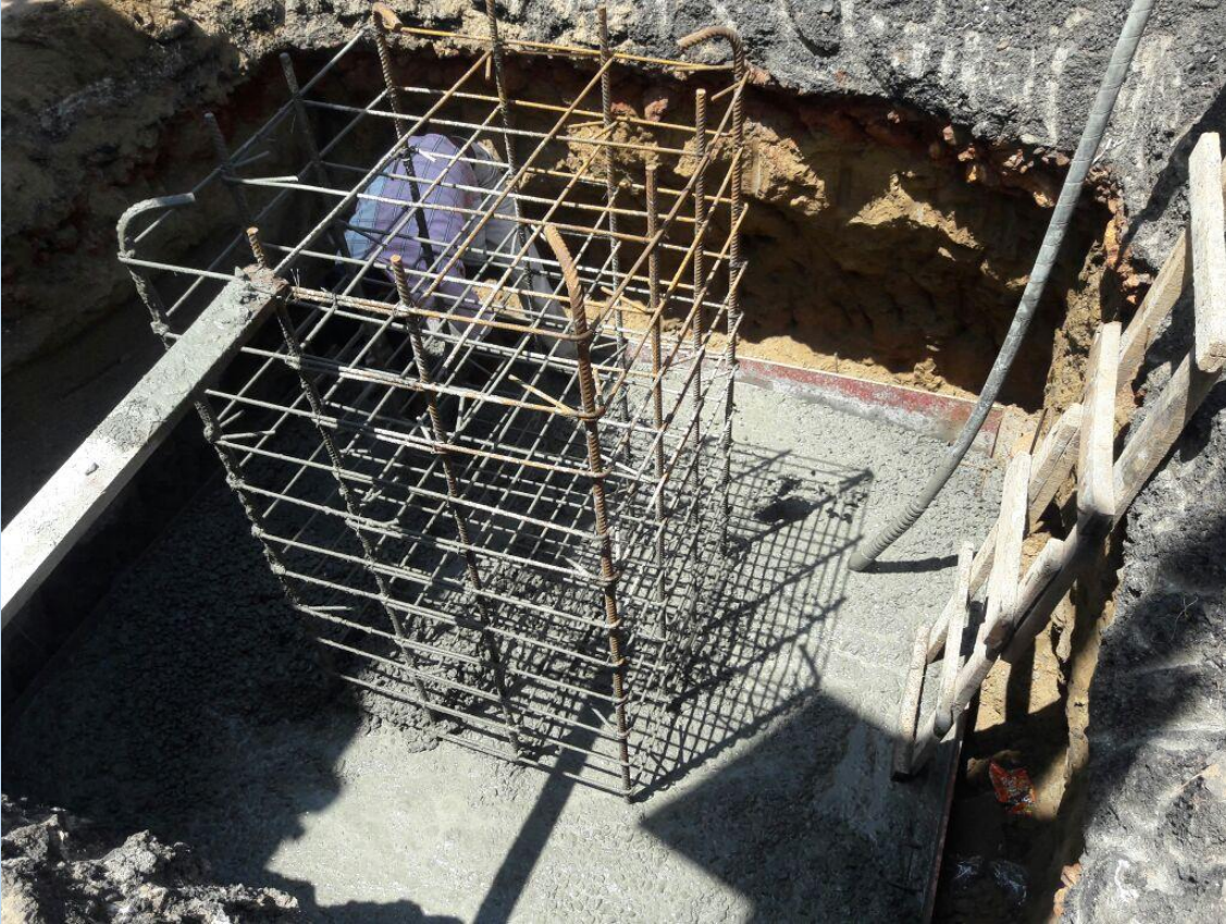
VMD Sub structure construction is in progress
