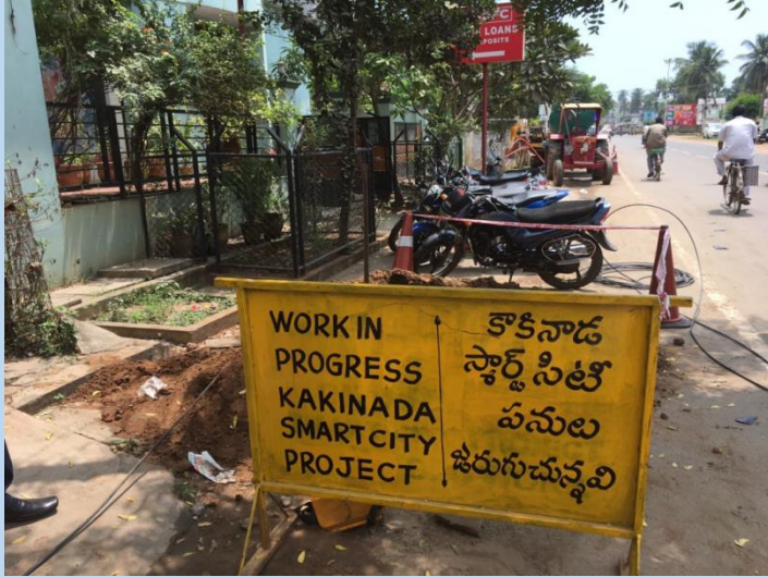
Optical fibre cable laying
