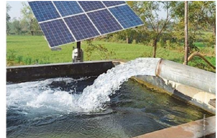
Solar Pump Installation
