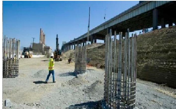
Pile Foundation Bridge Under PWD
