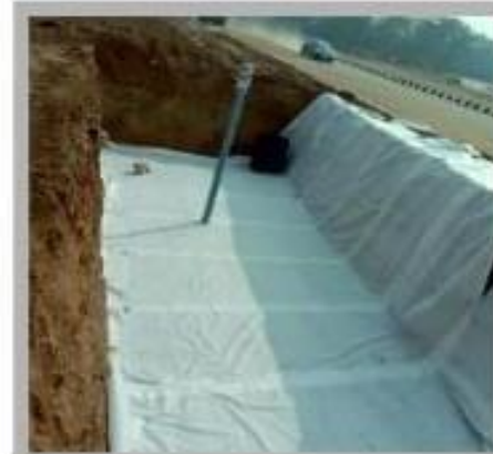
Laying of Geotextile
