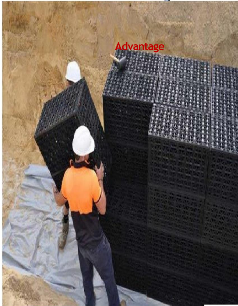
under the parking lot, at shopping centre (Storage capacity:6,600m 3 )
