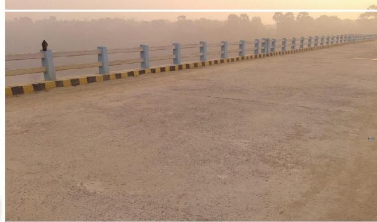
Bridge Construction (Pile Foundation & Well-Sinking Bridges)
