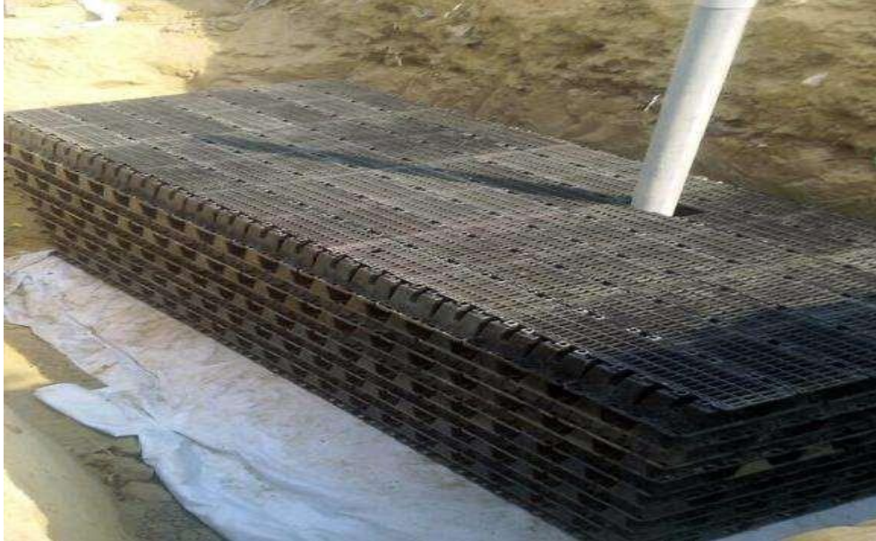
TYPICAL SECTION OF CROSS WAVE POLYMERS
