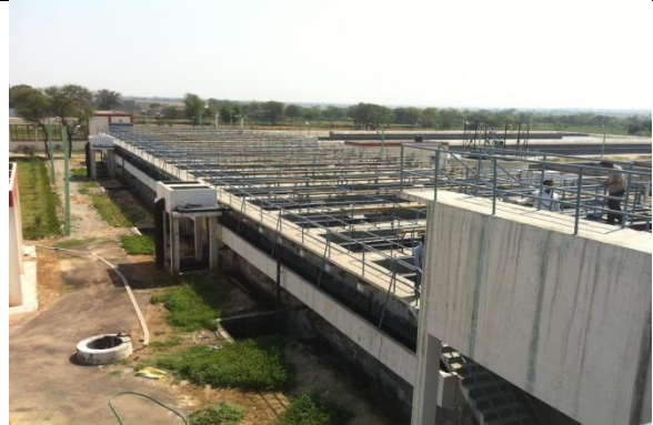
16 MLD UASB STP (yet to be fully commissioned)
