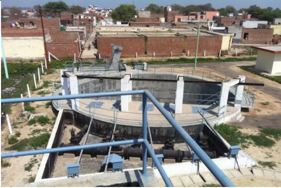
Kulu Ka Nagla MPS (newly constructed)
