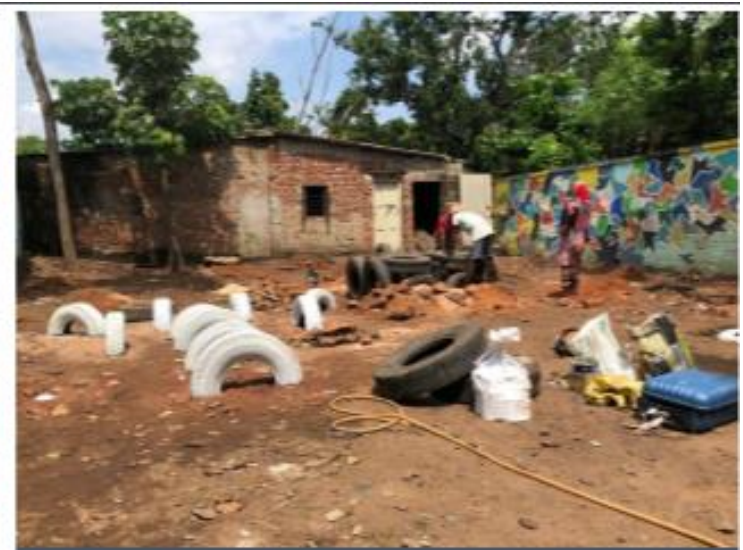
Building the play elements
