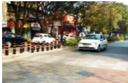
Raised Pedestrian Crossing
