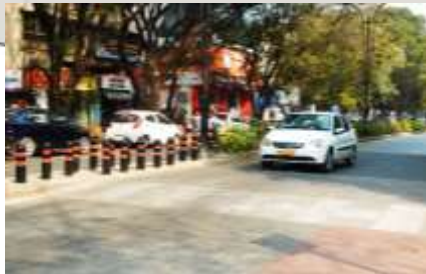
Raised Pedestrian Crossing
