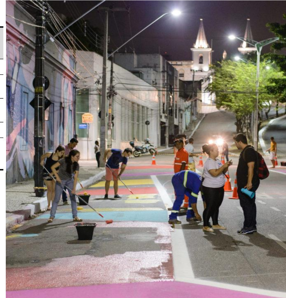
Photo: City contractors and local volunteers redesign the street to make it safer for people Source: NACTO
