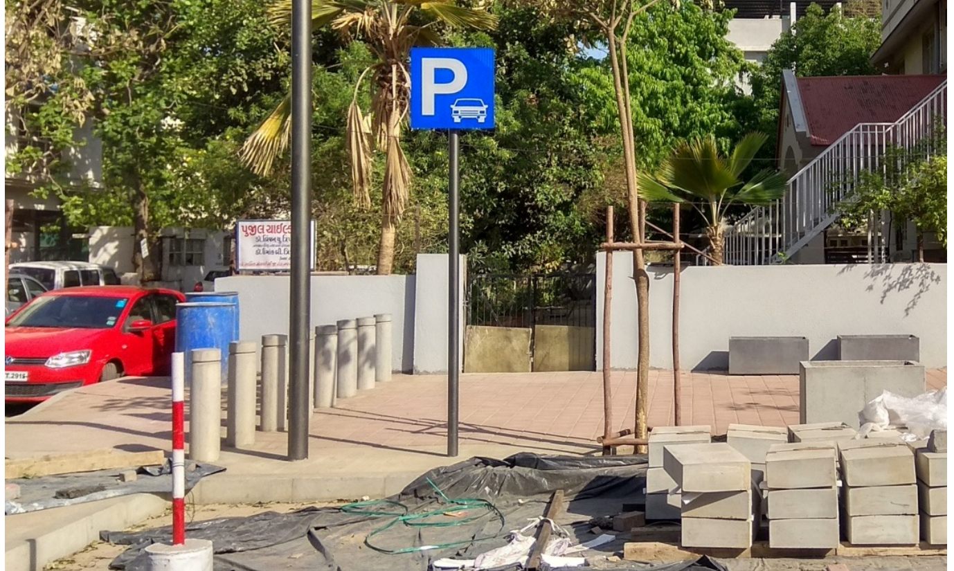
Installed Signage Pole
