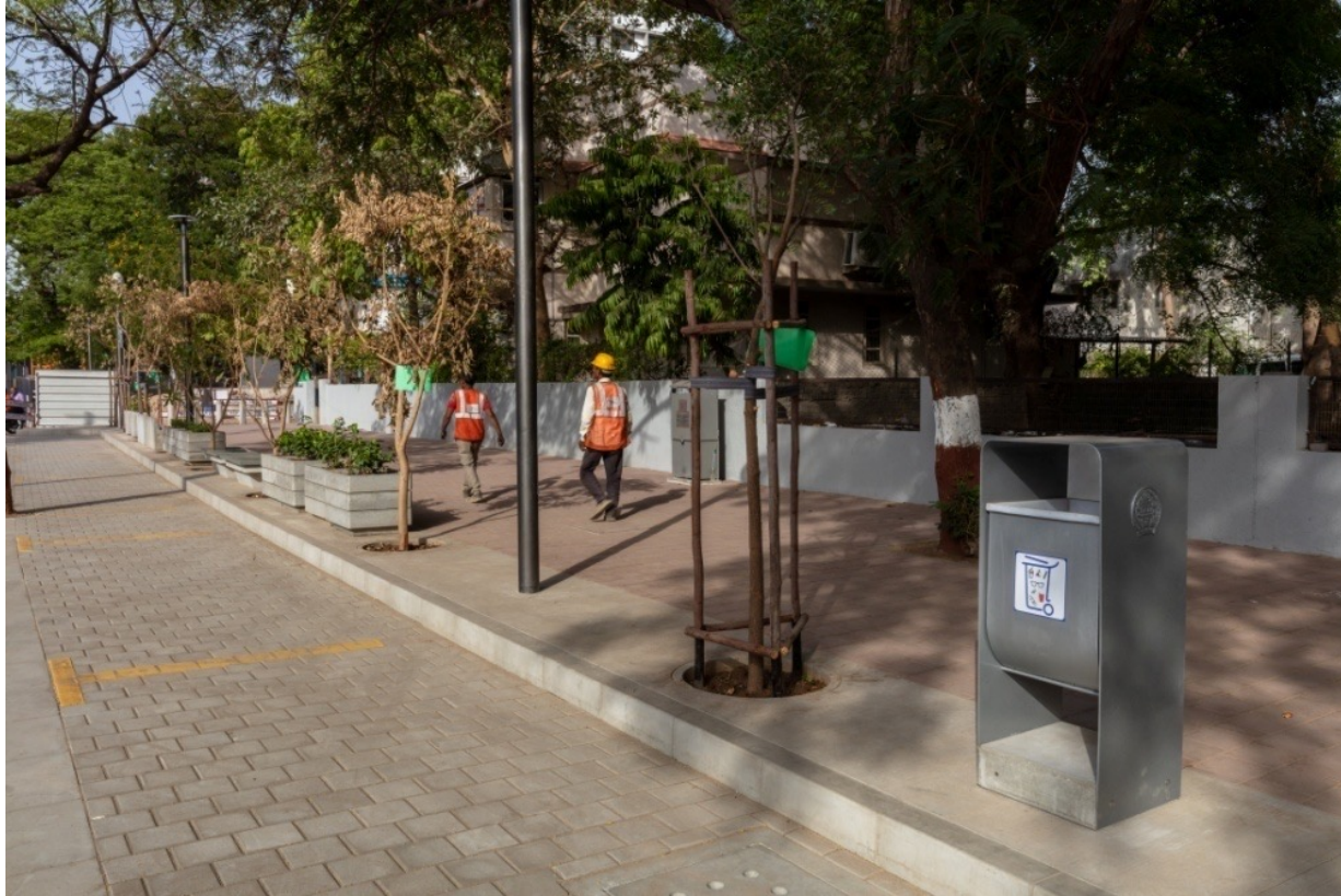
Installed Dustbins on Site
