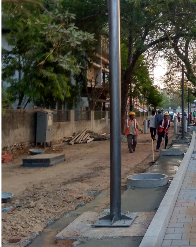
Installing Light Poles
