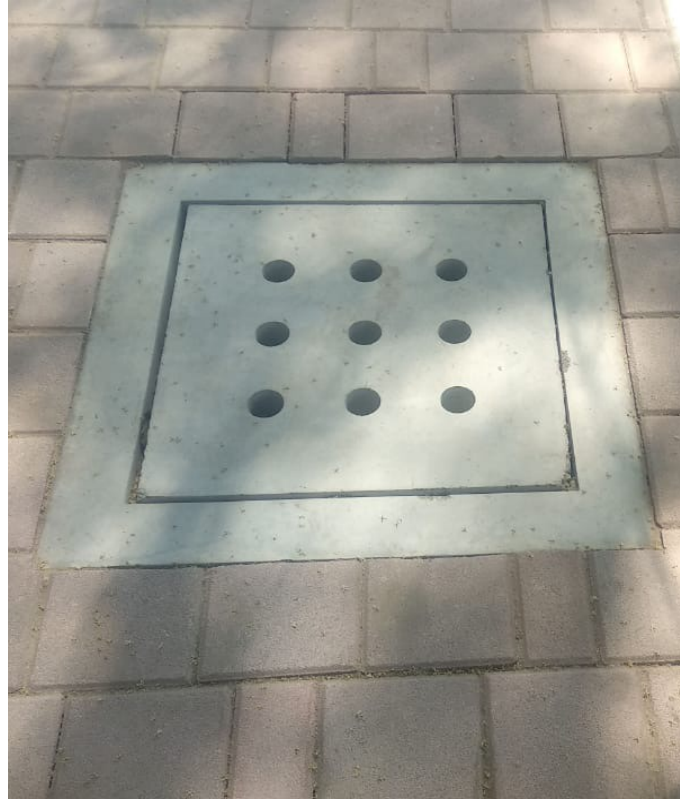
Proposed Drains Executed
