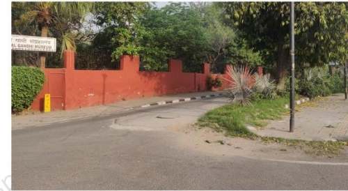
Figure 21. Access / Service lanes - open out onto the intersection. Crossings are discontinued at this point, endangering pedestrians.
