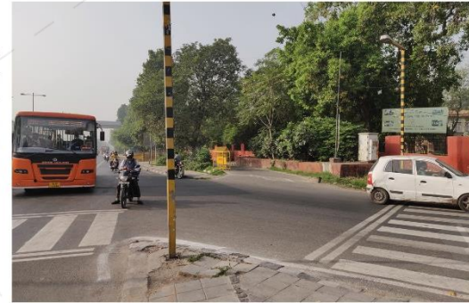
Figure 29. 02 poor quality of pedestrian refuge, lack of accessibility for the physically and visually challenged, access road opening up onto the intersection, and free left promoting speeding and rash driving.
