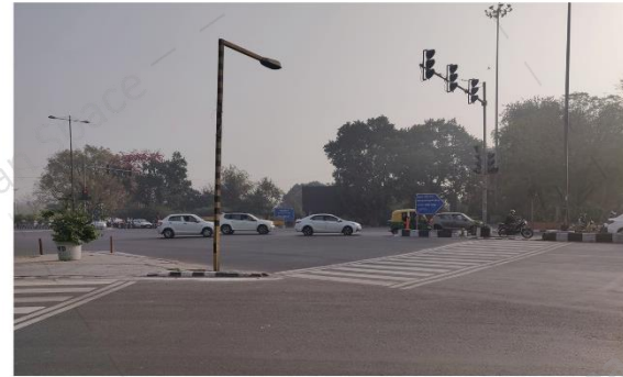
Figure 27. 01 photograph taken early in the morning, showing poorly designed pedestrian crossings, vehicular stop lines and signboards absent.
