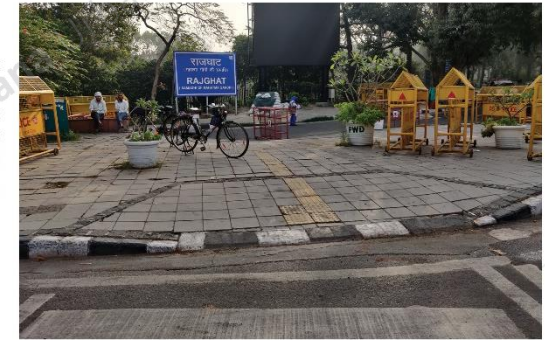
Figure 31. 05 curb cut designed for universal access but footpath is encroached with traffic barricades and potted plants.
