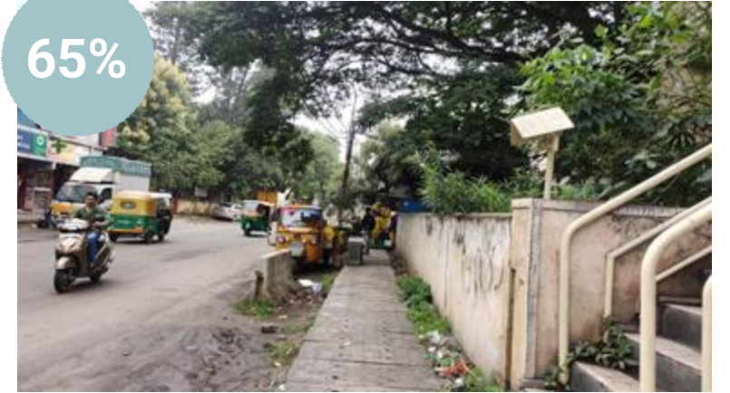
Narrow Uneven/ Discontinuous Footpath
