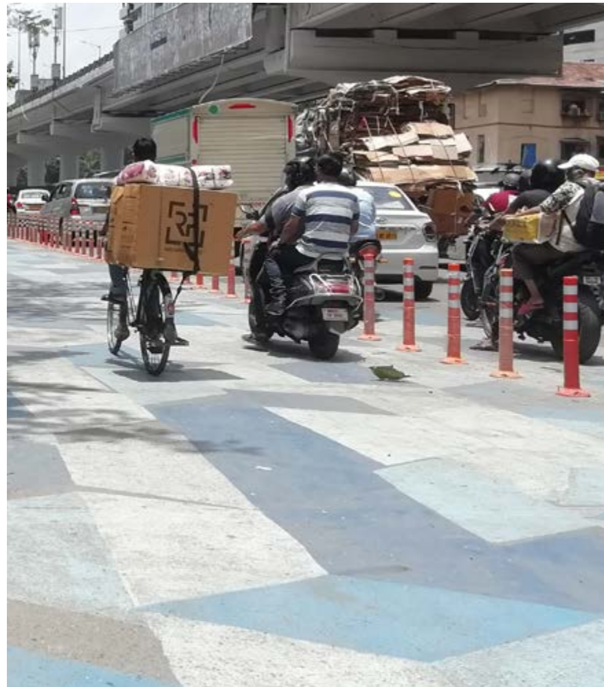
Creating of public realm using paint and bollards
