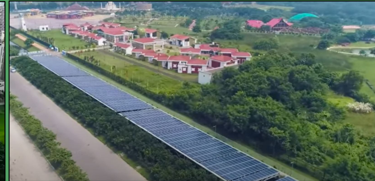
Canal Top Solar Panel in New Town
