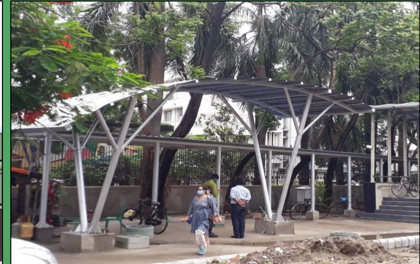
Fig 4. Ongoing Construction Work for Smart cycle stand
