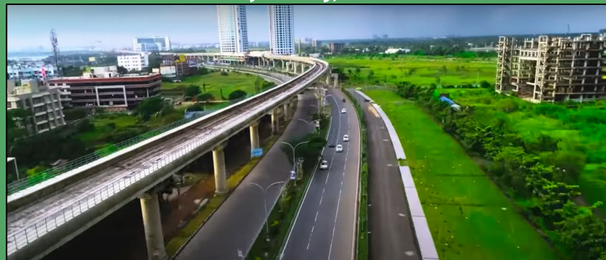
New Town- an over head utility-free zone
