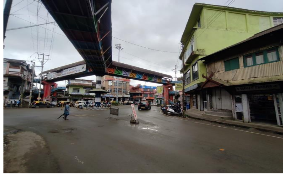
Unsafe intersection: Lack of traffic lights, heavy traffic
