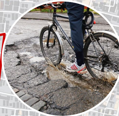
Poor road surface
