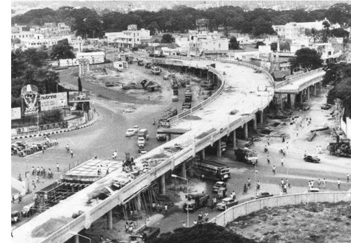
Construction of the Gemini Flyover, 1972 | Source: The Hindu Archives
