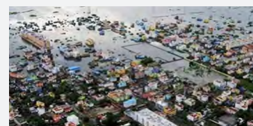
Aerial view of Chennai flooded | Source: PTI
