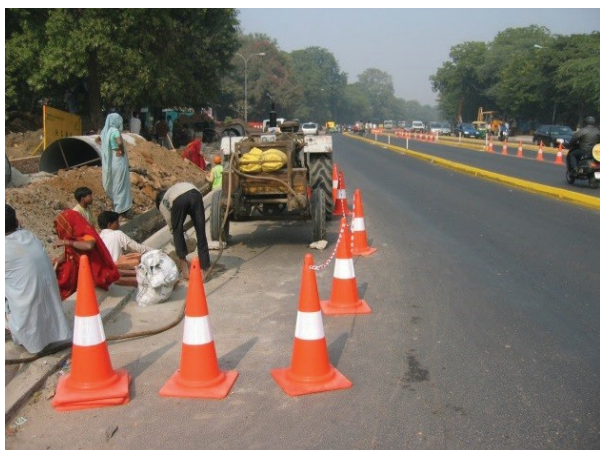
Figure 6.2: Supervision at the site Source: iTrans
