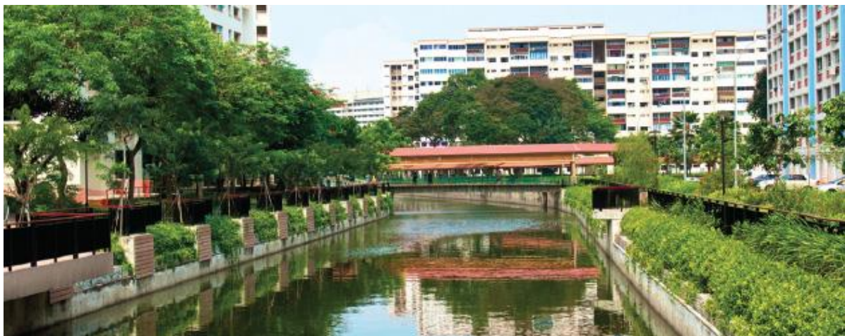
Figure 4.16: View of a water channel development
