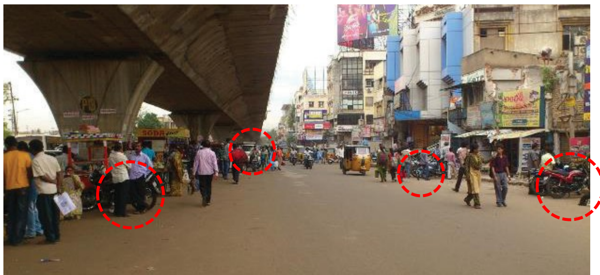
Figure 2.22: On-street parking in conflict with pedestrians beneath Telugu Talli Flyover
