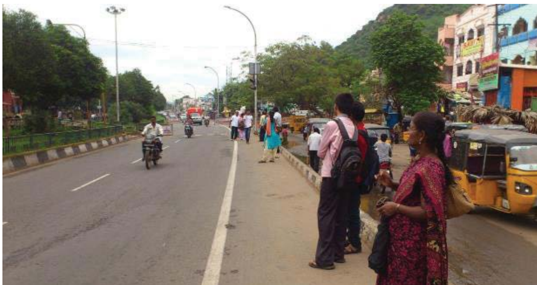
Figure 2.12: Inadequate bus stop facilities
