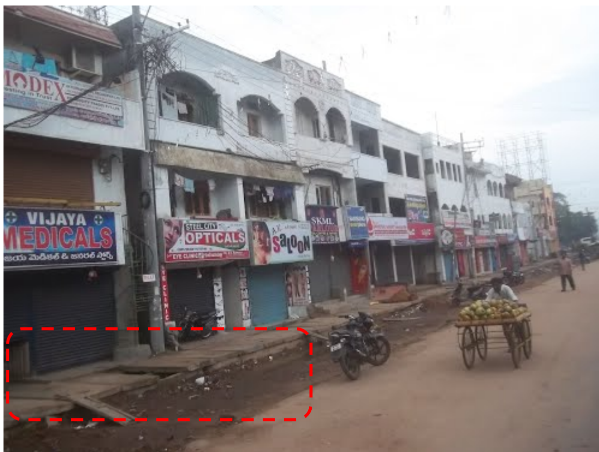
Figure 2.9: Drain covers on the left are unusable and unsafe as footpaths at Bowdra Ring Road near Balabharati Nagar Source: http://www.panoramio.com/photo/101174050
