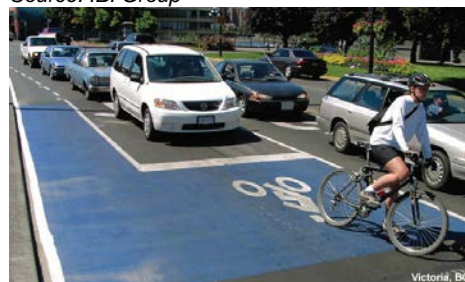
Figure 4.34: Paint marking of bicycle box at intersection, Vancouver BC
