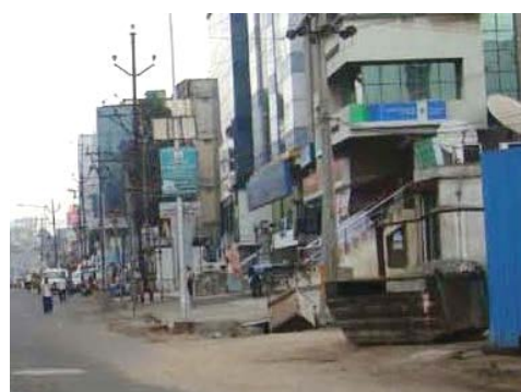
Figure 4.30: Haphazard and ill maintained footpath areas (Seven hill Jn. Road)
