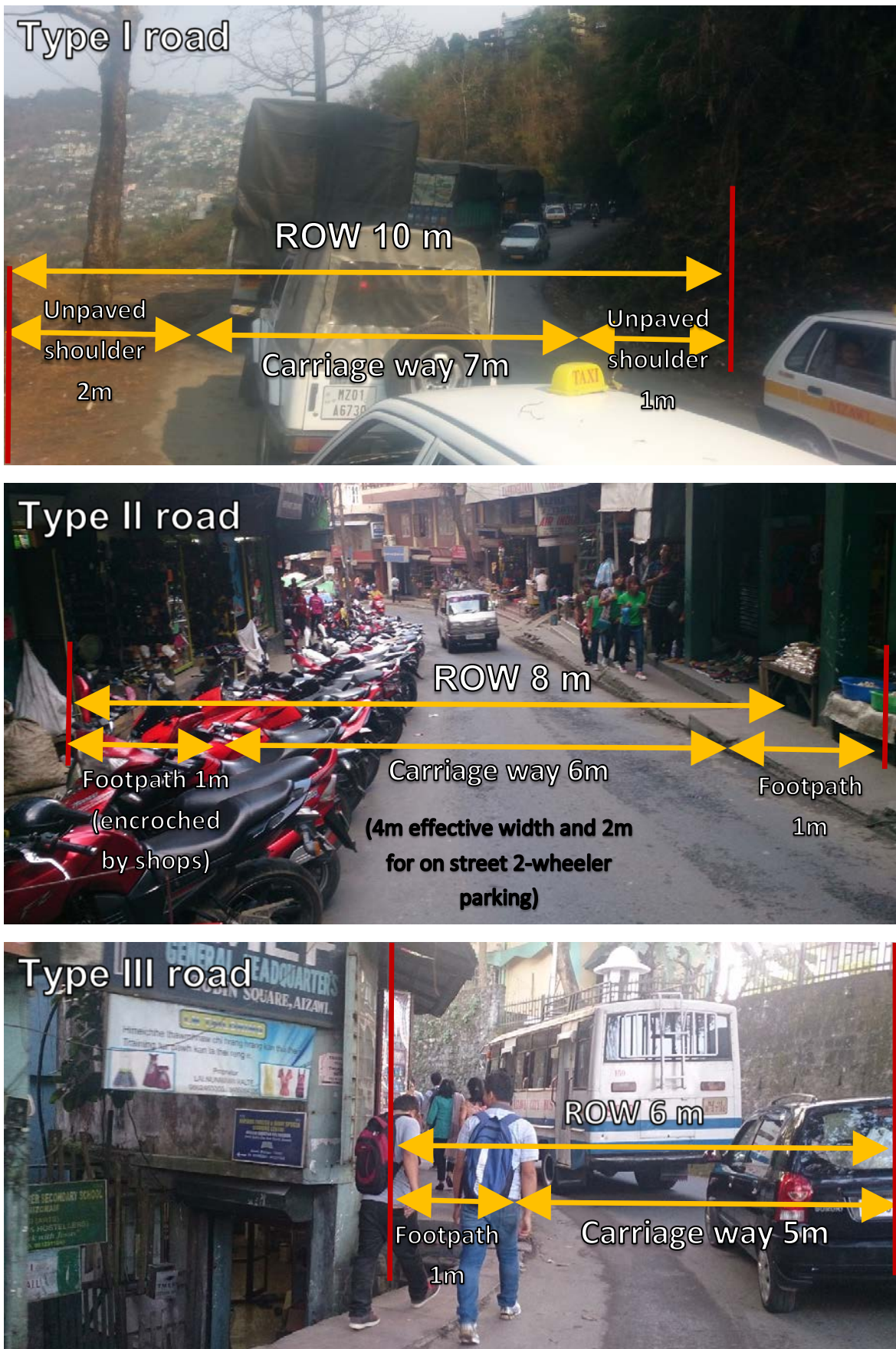
Figure 2.20: Typical cross section of Type I, II and III roads in Aizawl
