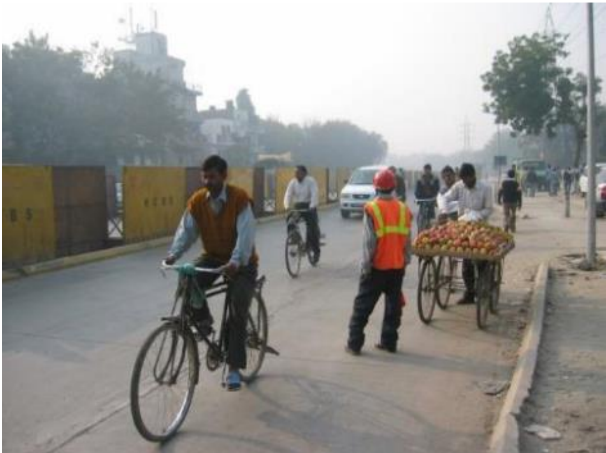
Figure 6.2: Traffic diversion and manned supervision during construction
