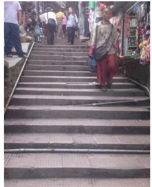
Existing condition of public stairs in Aizawl
